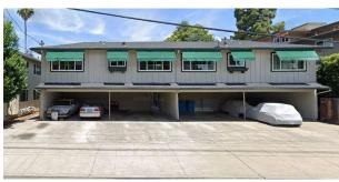
Figure 1 Example of a four-unit, soft-story building
