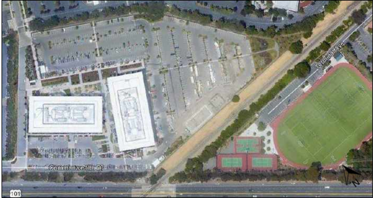
Figure 1. Existing project site.
