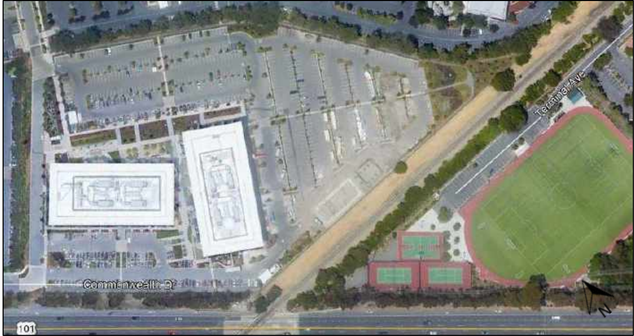
Figure 1. Existing project site.
