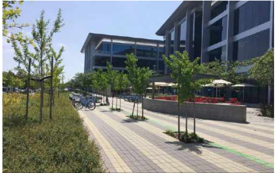
B. View of Buildings 1 and 2 Facing East.
