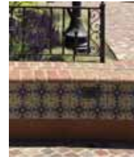
Seat Wall and Ornamental Fence
