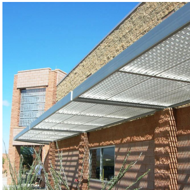
METAL AWNING W/ AMETCO "GROTTO" PANELS, PTD. ARCHITECTURAL BRONZE 8
