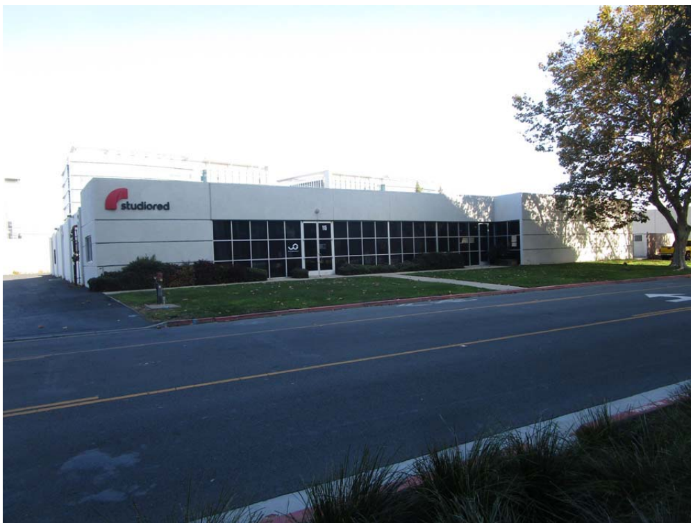
Southwest elevation (front view) of the building at 115 Independence Drive
