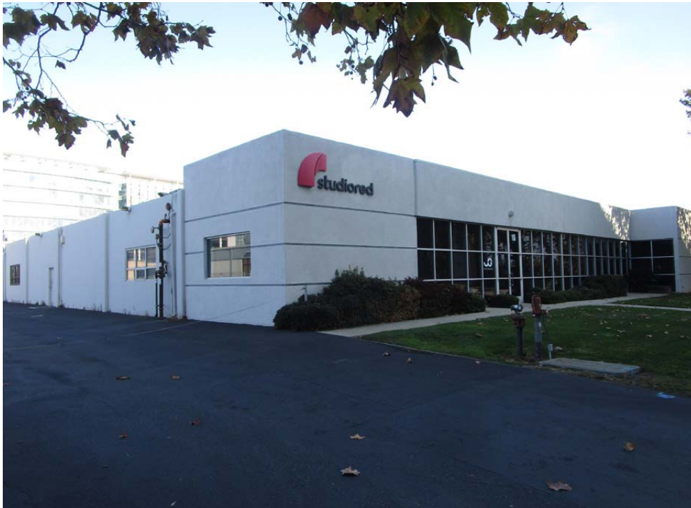
Southwest and northwest elevations (front and left sides) of the building at 115 Independence Drive
