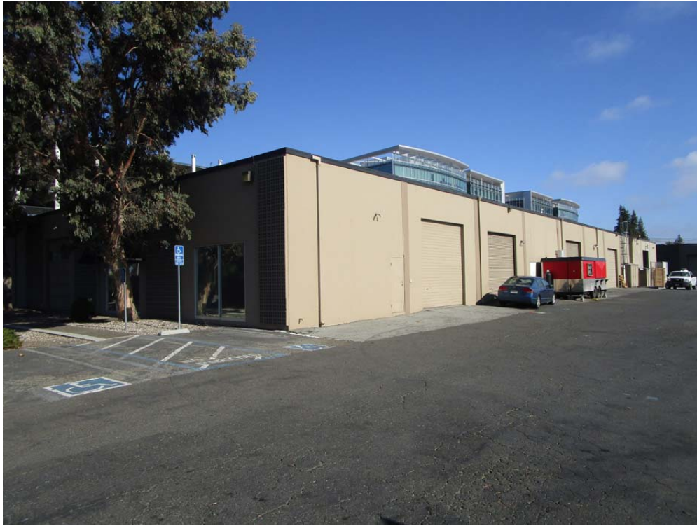
Southwest elevation (rear view) of the building at 104 Constitution Drive
