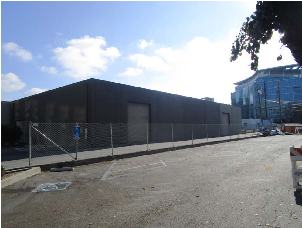
Northwest elevation (right side) of the building at 110 Constitution Drive as seen from the parking lot at 104 Constitution Drive
