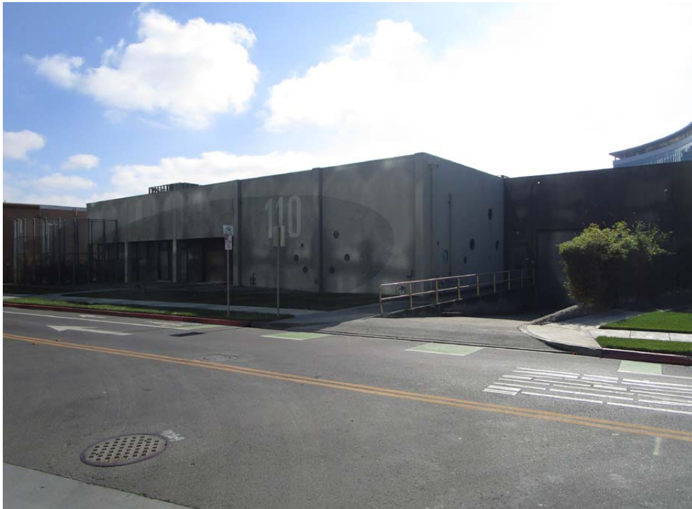
Northeast elevation (front view) of the existing building at 110 Constitution Drive
