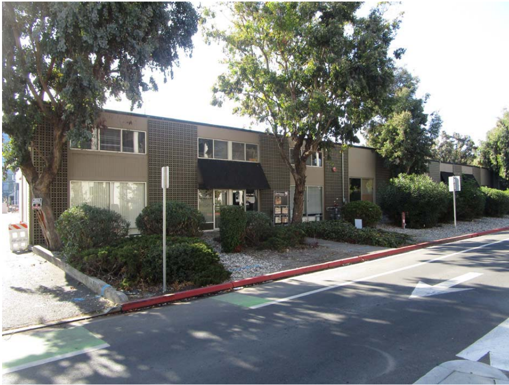
Northeast elevation (front view) of the existing building at 104 Constitution Drive
