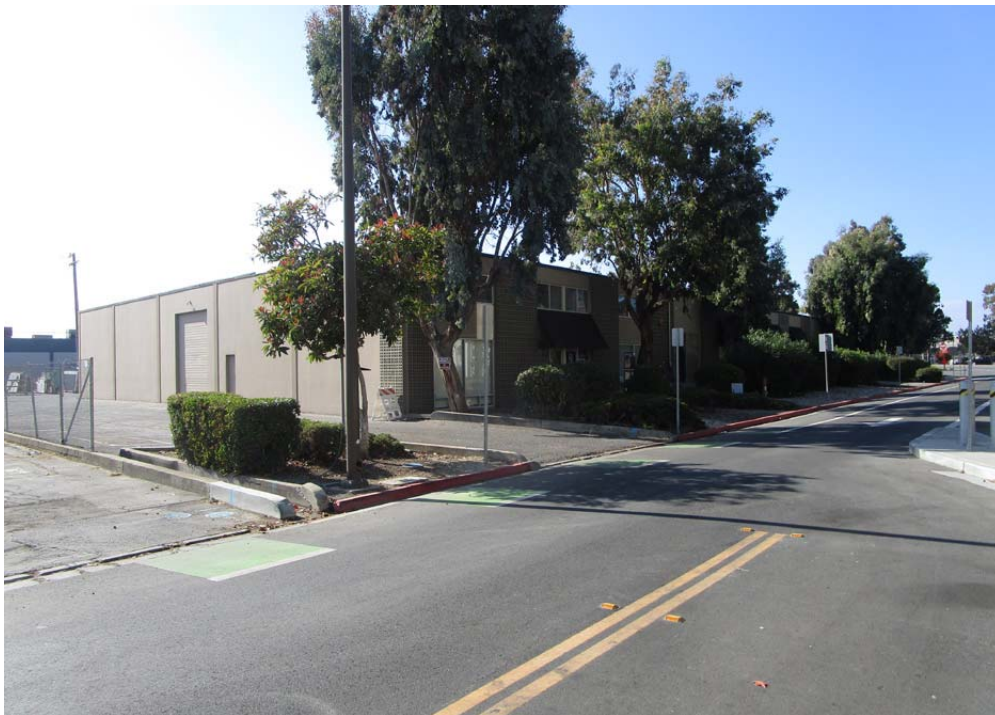
Northeast and southeast elevations (front and left sides) of the building at 104 Constitution Drive
