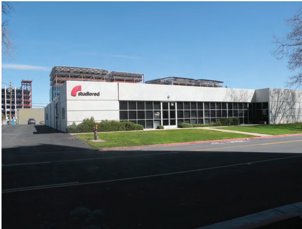
Photo 1: Existing building at 115 Independence Drive, as seen from Independence Drive
