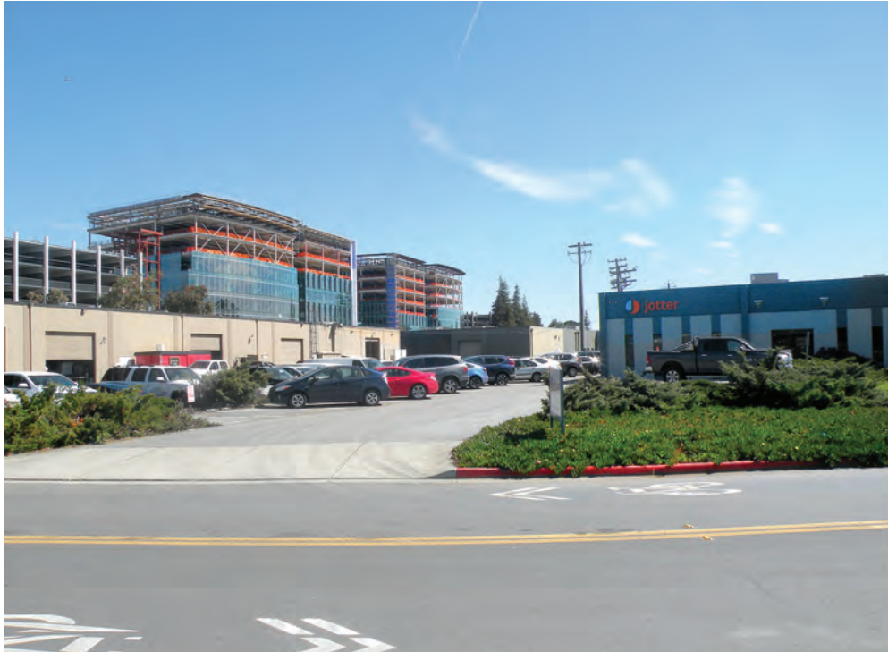
Photo 3: Photo of Constitution Site of Menlo Gateway Project, as seen from Independence Drive, north of the project site
