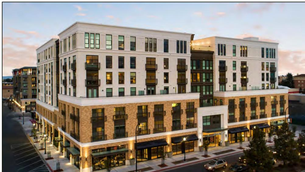
**Overview:** Huxley Apartments is an 8-level, 137-unit multi-family residential development entailing one level of underground parking, one level of above ground parking, and six levels of for-rent apartments, located within the Downtown Precise Plan Area.
