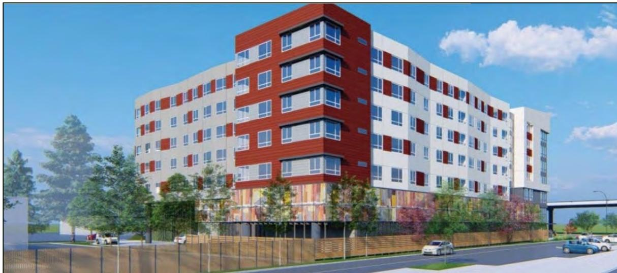
**Overview:** The project proposes to demolish an existing 19,440 square-foot, one-story industrial building and construct a 176-unit multi-family housing development within a seven-story building (five levels of housing on top of two levels of podium parking). The property is located directly next to the Lawrence Caltrain Station. The 1178 Sonora Court community is being developed by MidPen Housing in partnership with the City of Sunnyvale.
