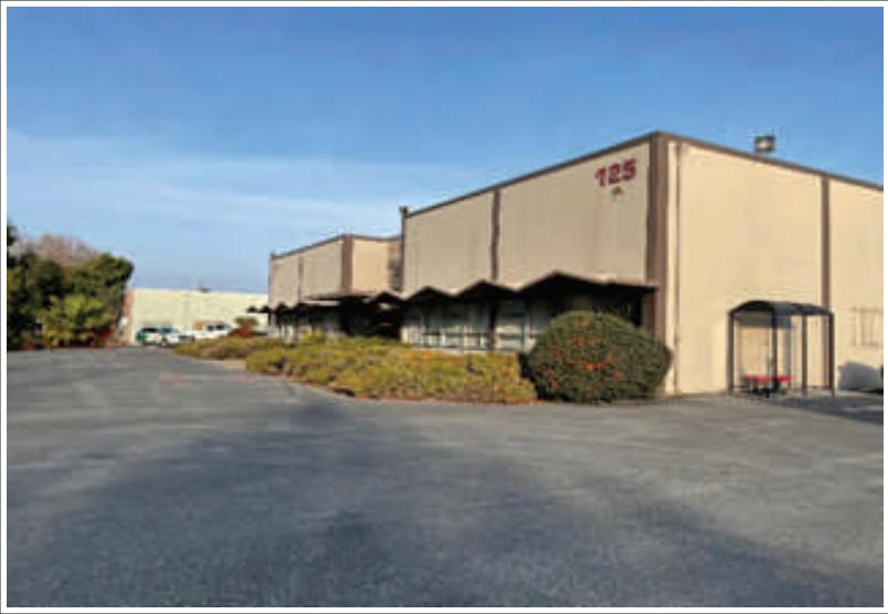
Photo 5: Existing building on the project site. Facing northwest.
