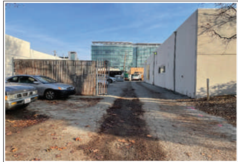
Photo 8: Existing parking, driveways, and fence structures surrounding existing buildings of the project site. Facing south.
