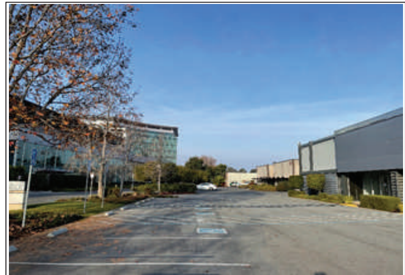
Photo 4: Buildings and parking areas along southern boundary of the project site. Facing west.
