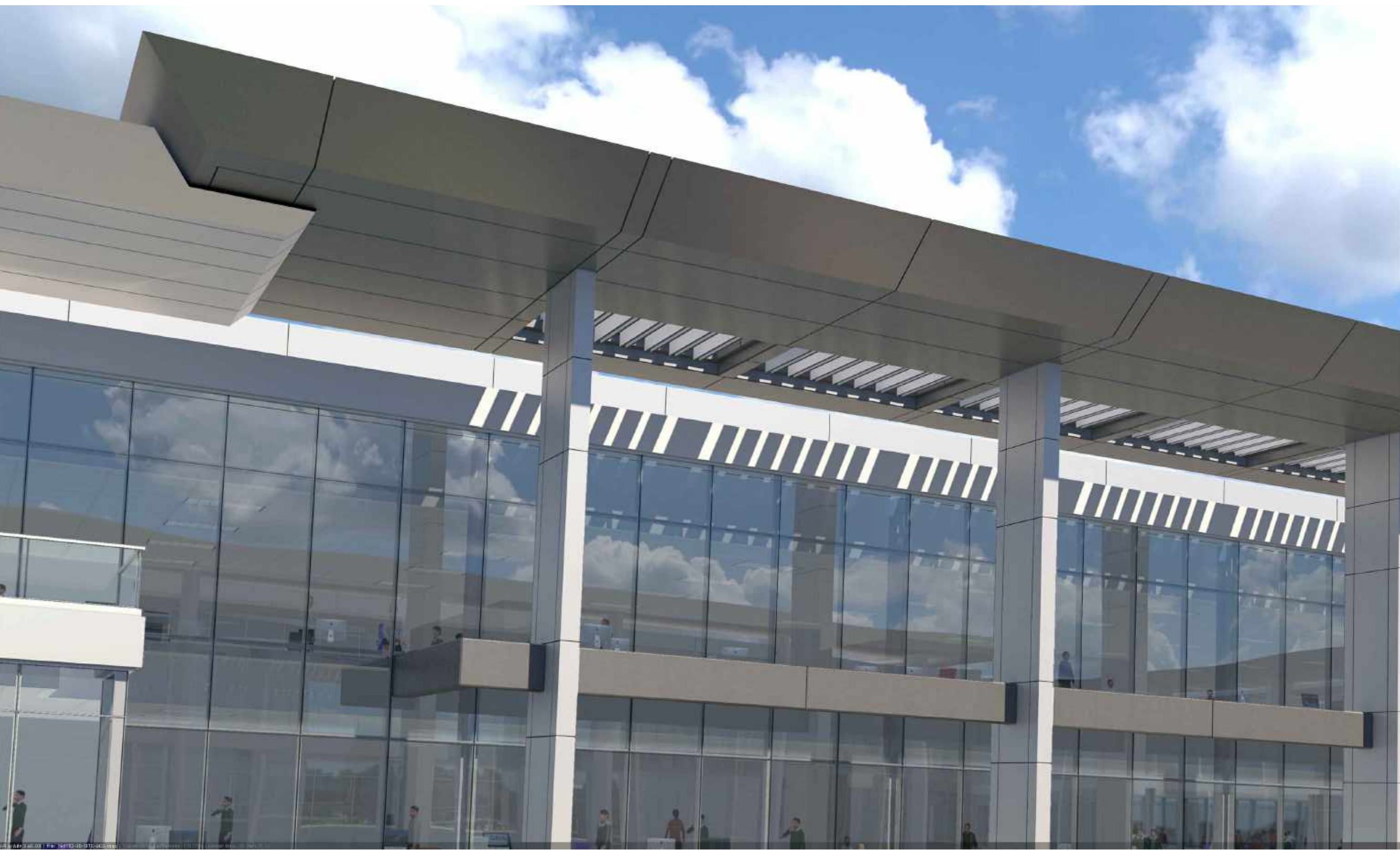
2 DETAIL VIEW OF ALUMINUM COMPOSITE METAL CANOPY AND LOUVERS ON SOUTH FACADE
