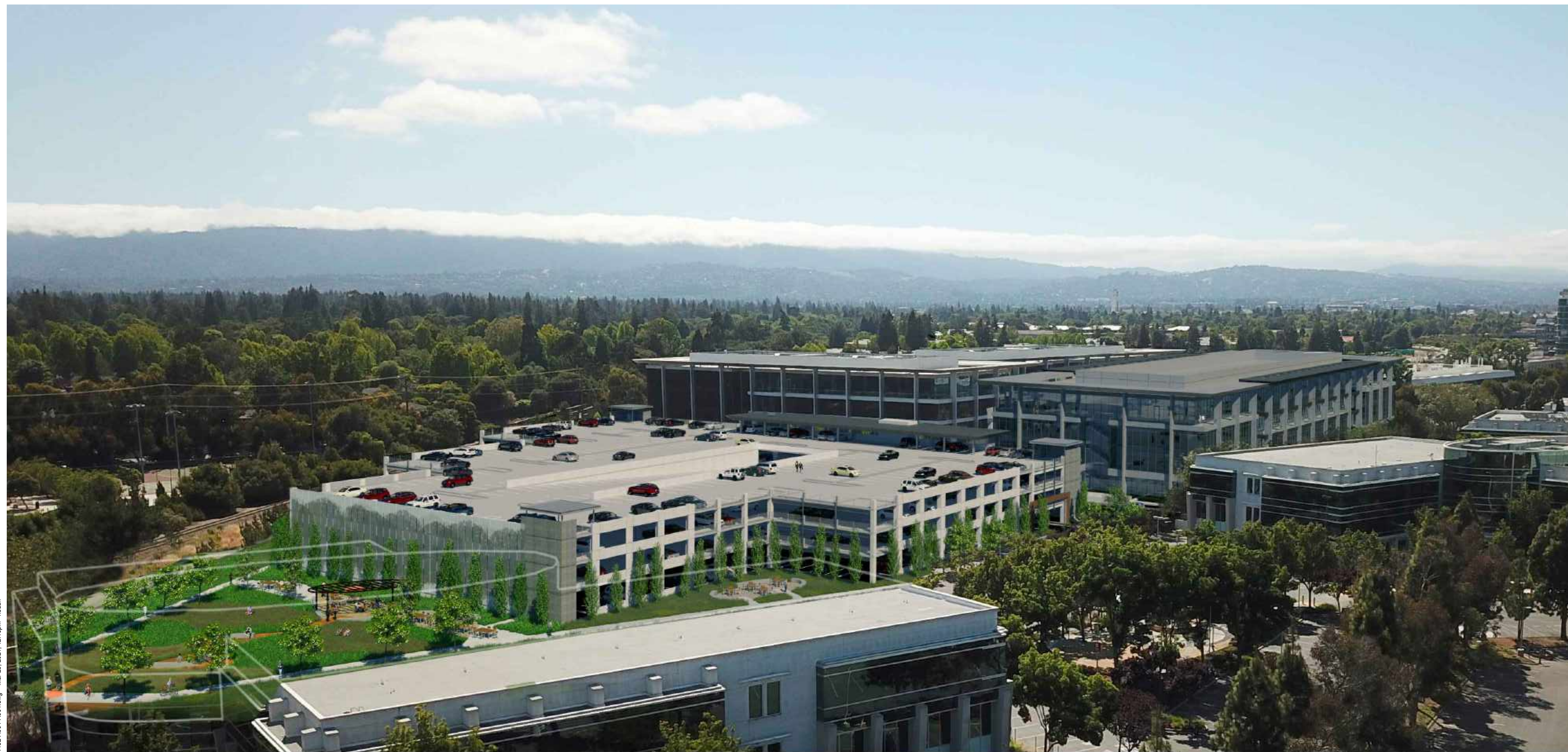
2 AERIAL VIEW FROM NORTH OF SITE LOOKING SOUTH
