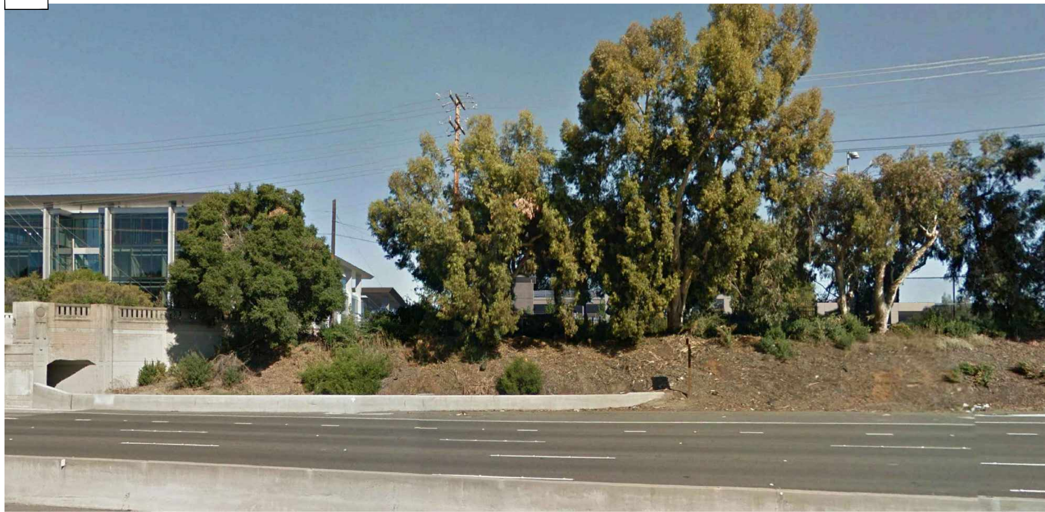
2 VIEW FROM 101 BAYSHORE FREEWAY LOOKING NORTH EAST
