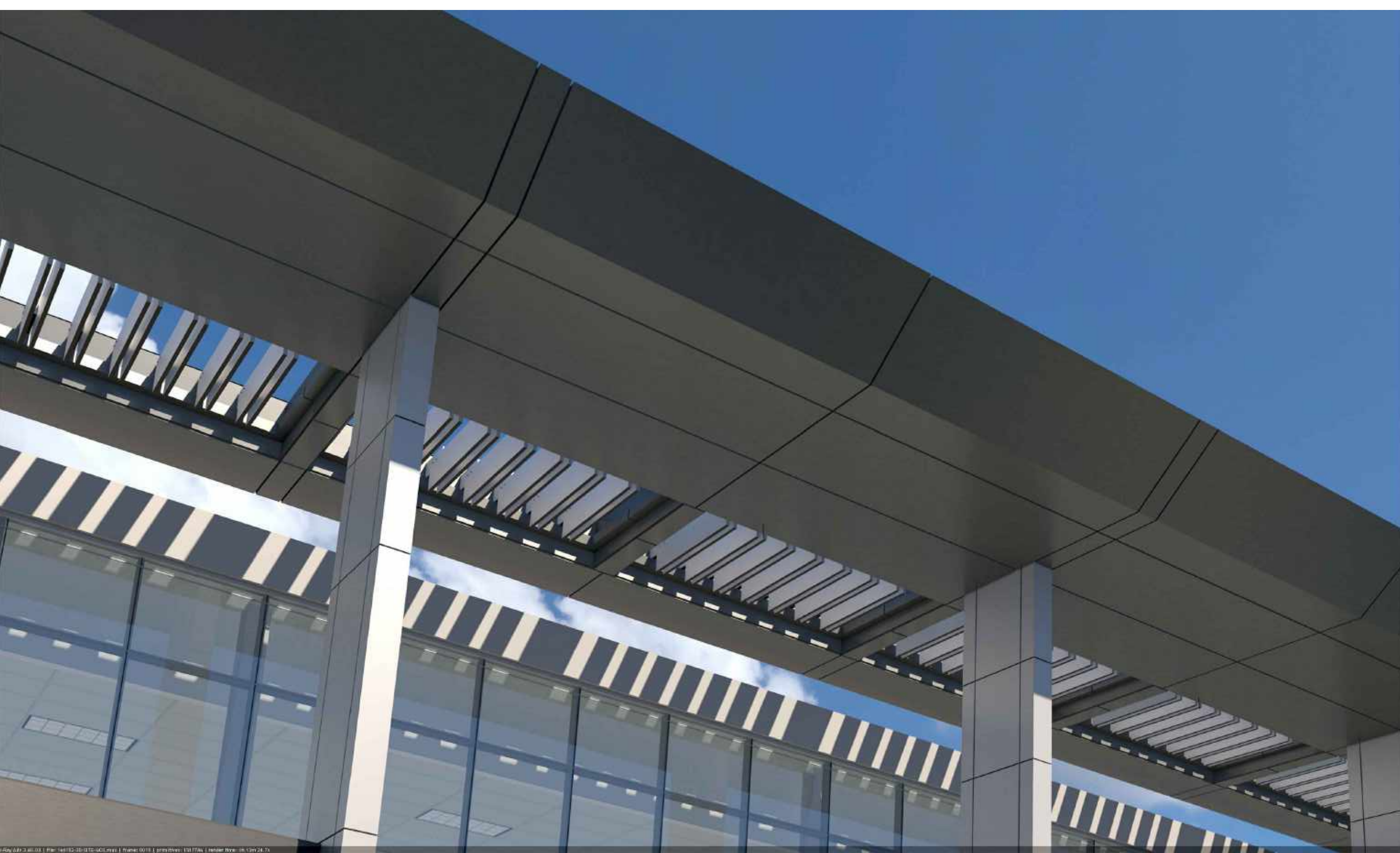
1 DETAIL VIEW OF ALUMINUM COMPOSITE METAL CANOPY AND LOUVERS ON SOUTH FACADE
