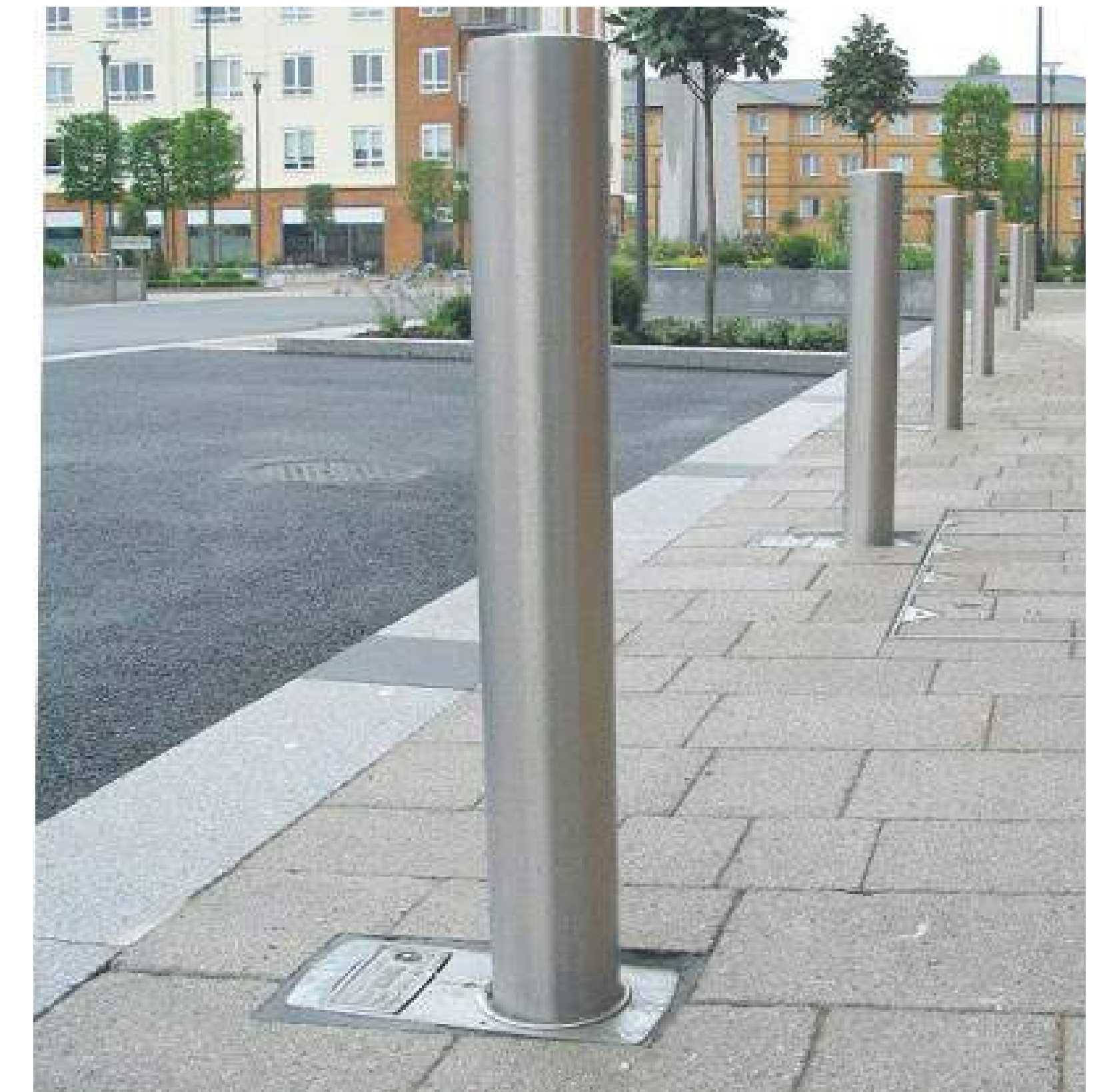
Retractable Bollard Example
