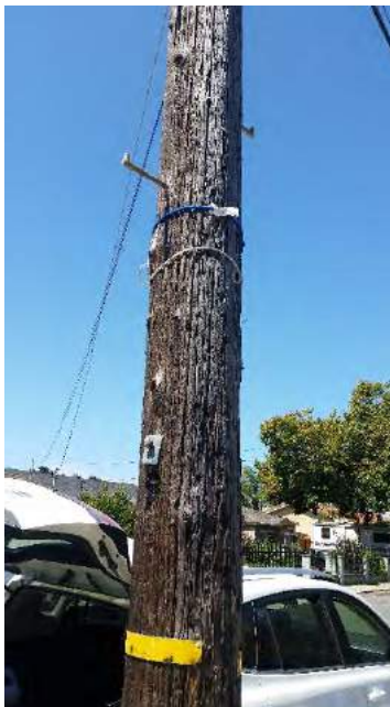
Looking Southwest along Alberni Avenue.
