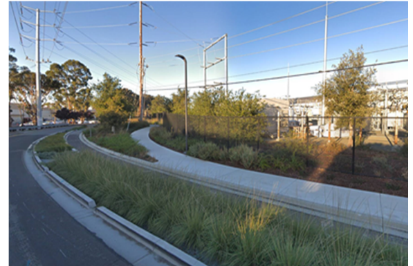
Figure 1-4 Stormwater planter at Chilco Street, Menlo Park
