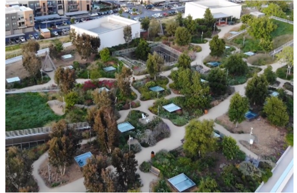
Figure 1-9 Green Roof, Facebook, Menlo Park
