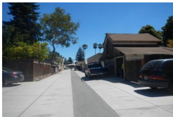
Figure 1-7 Infiltration trench, San Jose
