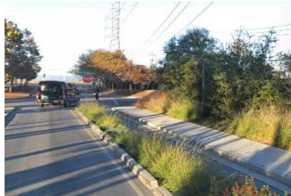
Example 3: Green Street (Chilco Street, Menlo Park)
