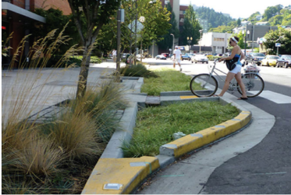
Figure 1-2: Stormwater curb extension example
