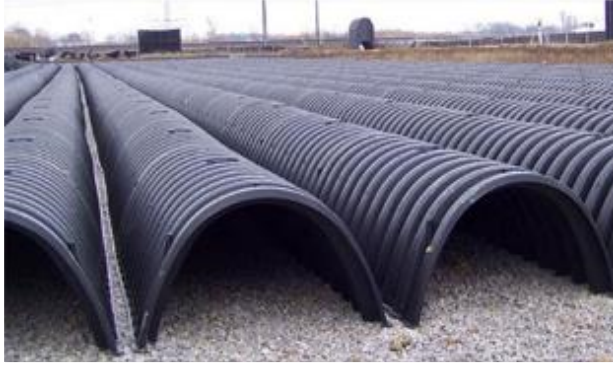
Example 1: Regional Stormwater Capture (subsurface infiltration)
