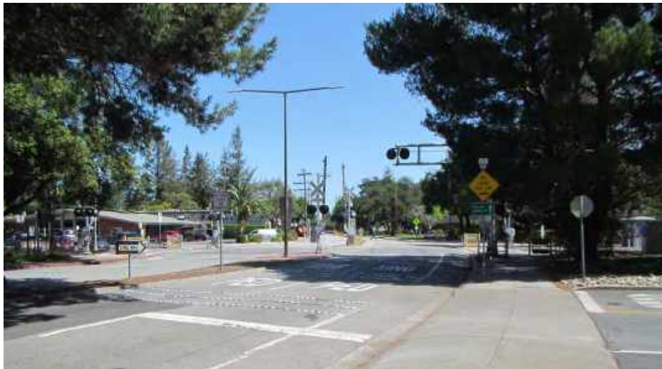
Figure 2. Ravenswood Avenue Rail Crossing, facing East
