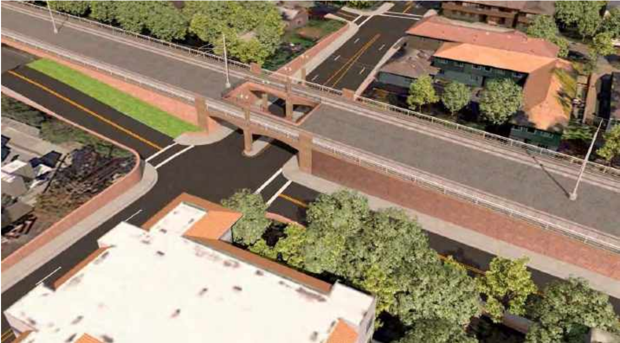
Figure 10 - Alternative C, Looking NE at Glenwood Avenue
