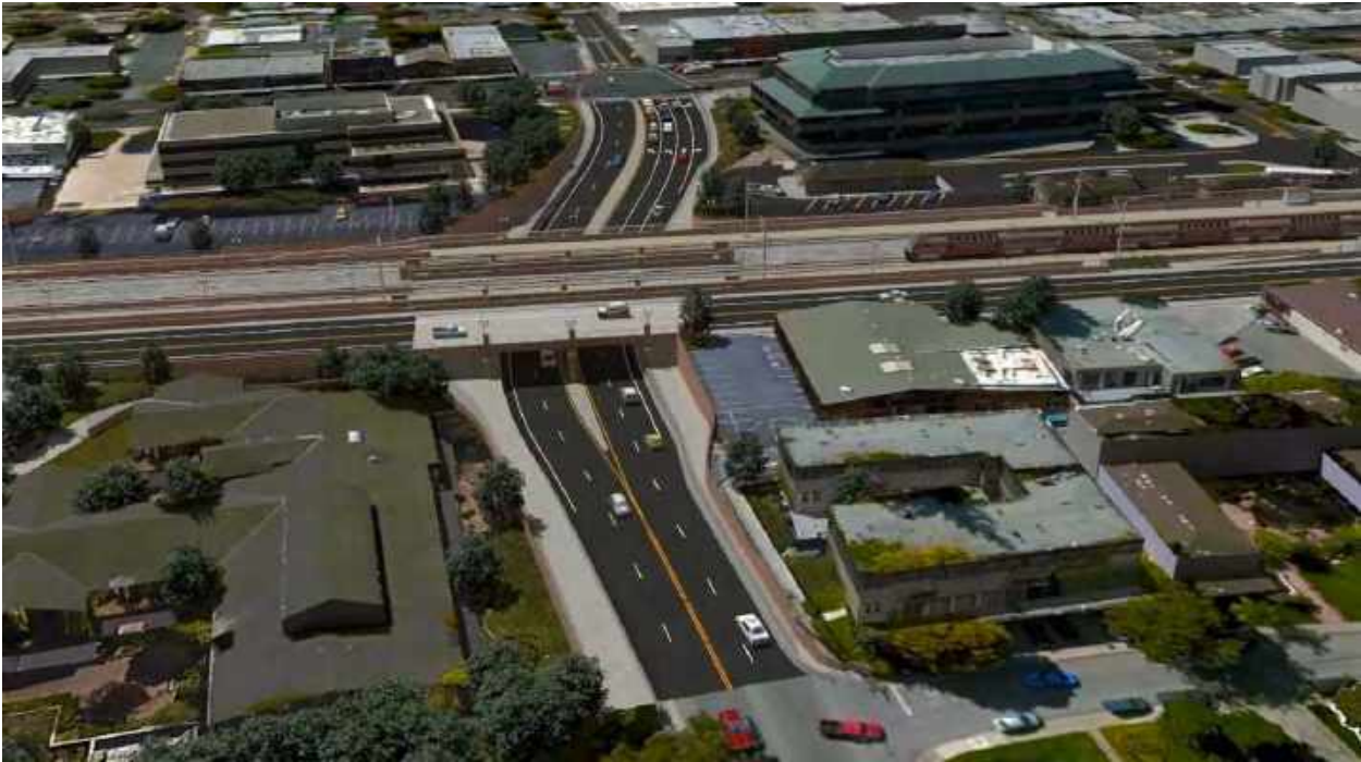
Figure 7 - Alternative A, Ravenswood Avenue, Looking West from Noel Drive
