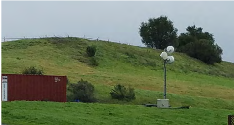
Photo 1. Steep Reservoir Embankment from the Southwest
