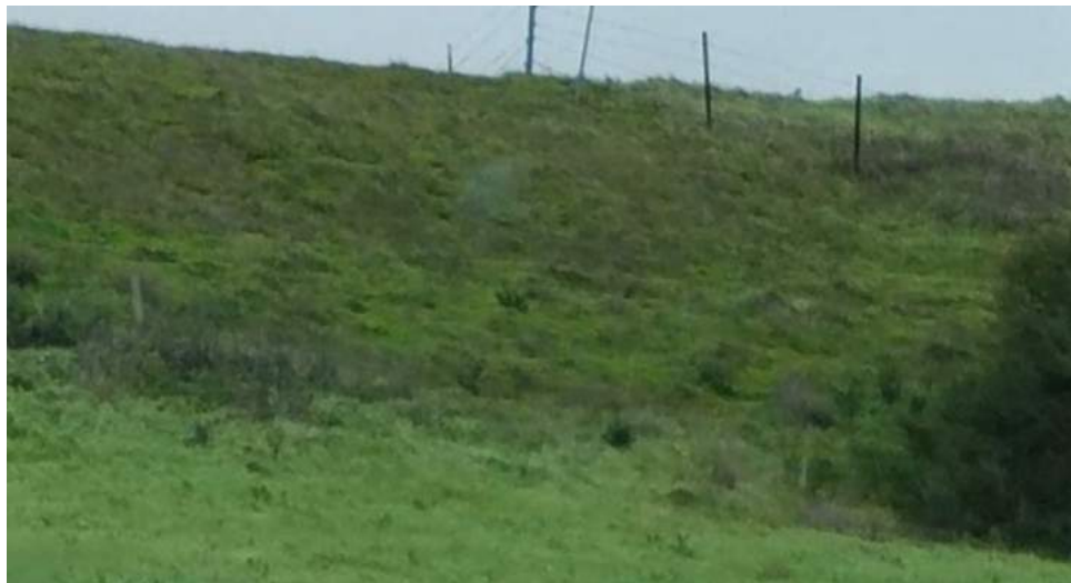
Photo 2. Closer view steep reservoir embankment
