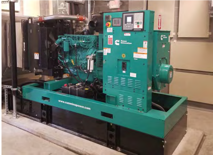
Photo 3. Diesel driven emergency generator at the Sharon Heights pump station. Fuel storage in the base of the unit limits capacity.
