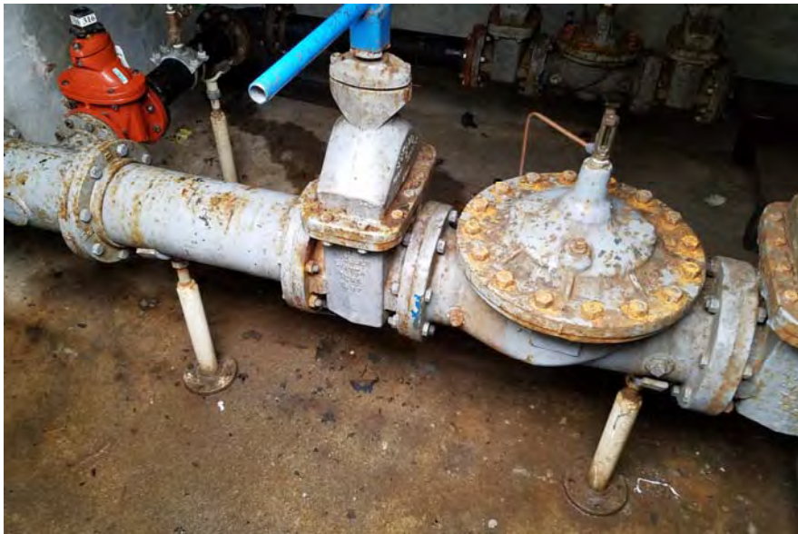
Photo 4. PRV Vault – Vertical pipe bracing not anchored to the floor; no horizontal bracing.
