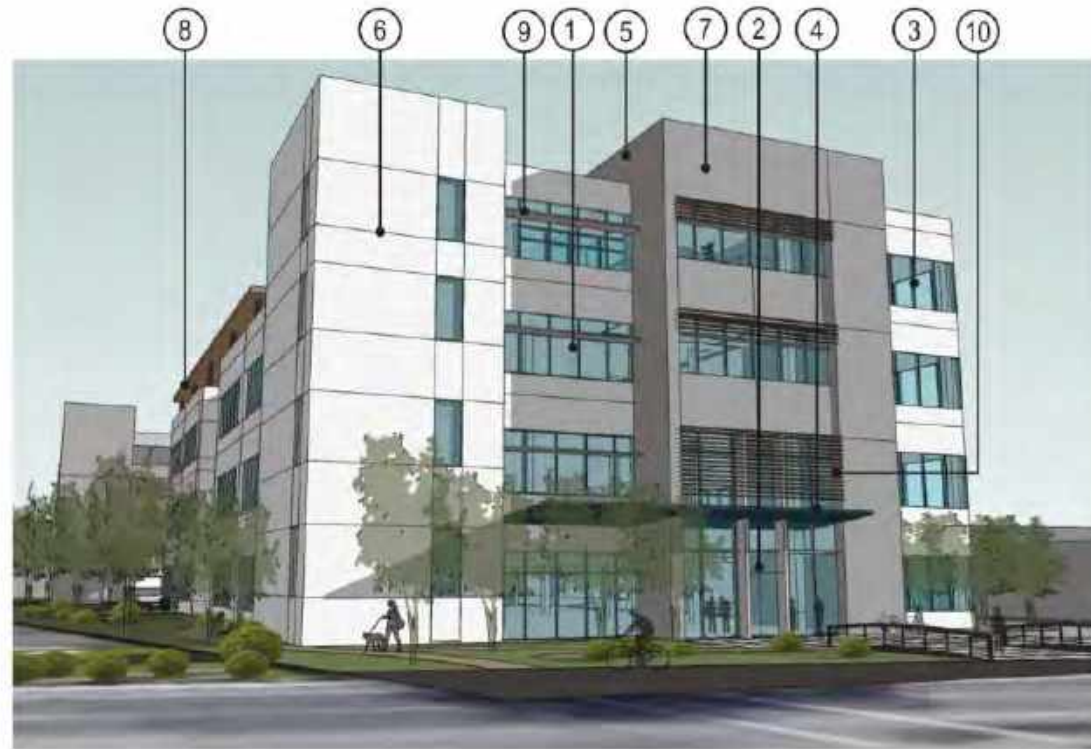
② GLASS (LOBBY), LOW-E, CLEAR DOUBLE GLASS (BIRD SAFE GLASS)
