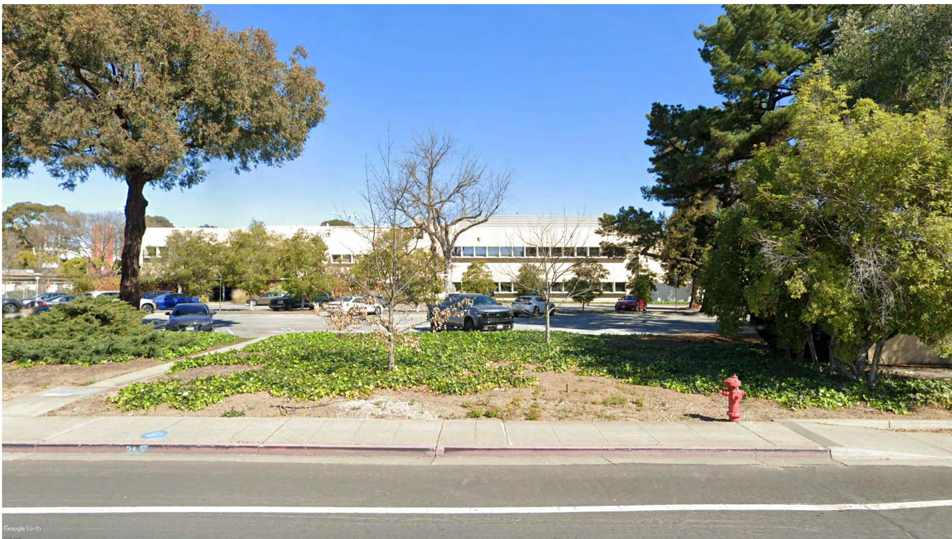
VIEW ON LAUREL TOWARD EAST
