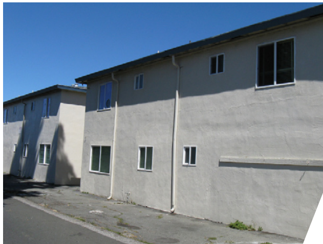
Additional parking and access through alleyway in rear
