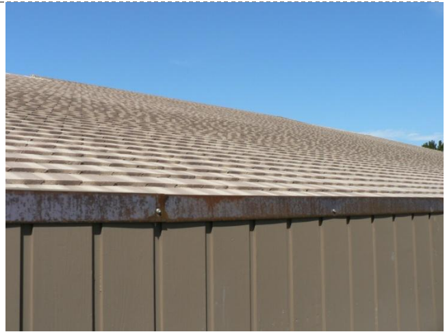
Figure 21 shows a view of the Gymnastics building rooftop
