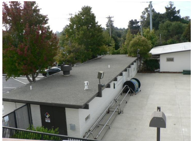
Figure 12 shows the roof of the pool house, Section 10
