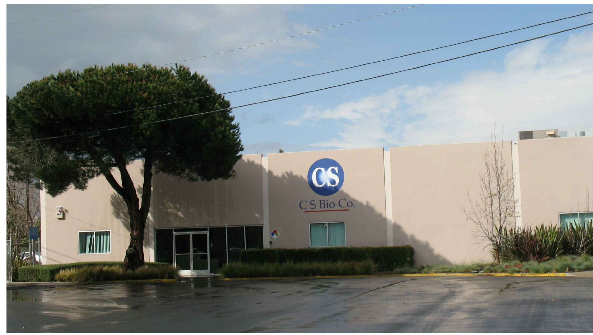
3 VIEW OF EXISTING CONCRETE BUILDING FROM KELLY COURT
