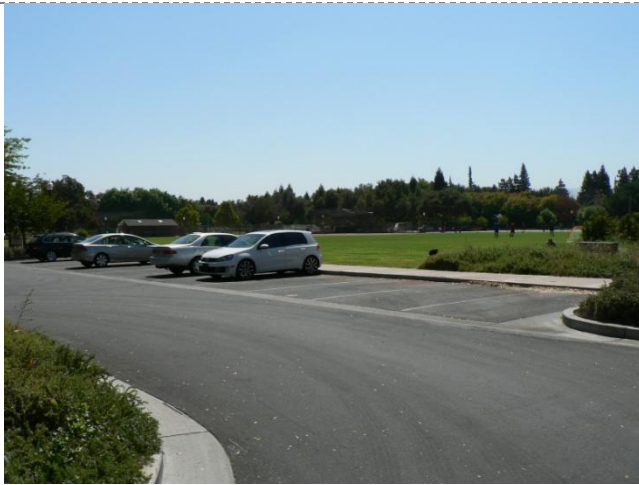
Figure 20 shows a view of Section 4 carport area
