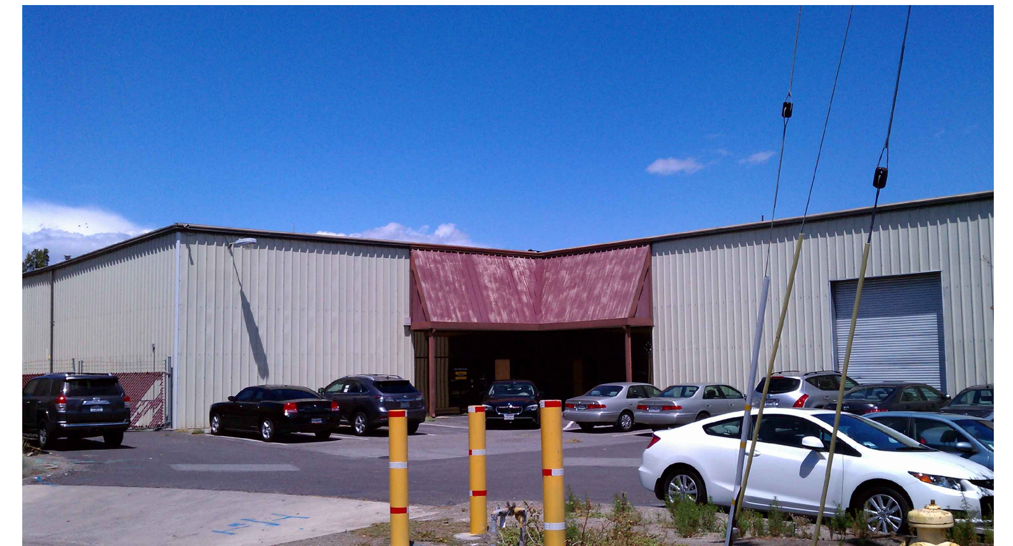
2 VIEW OF BACK OF INDUSTRIAL BUILDING
