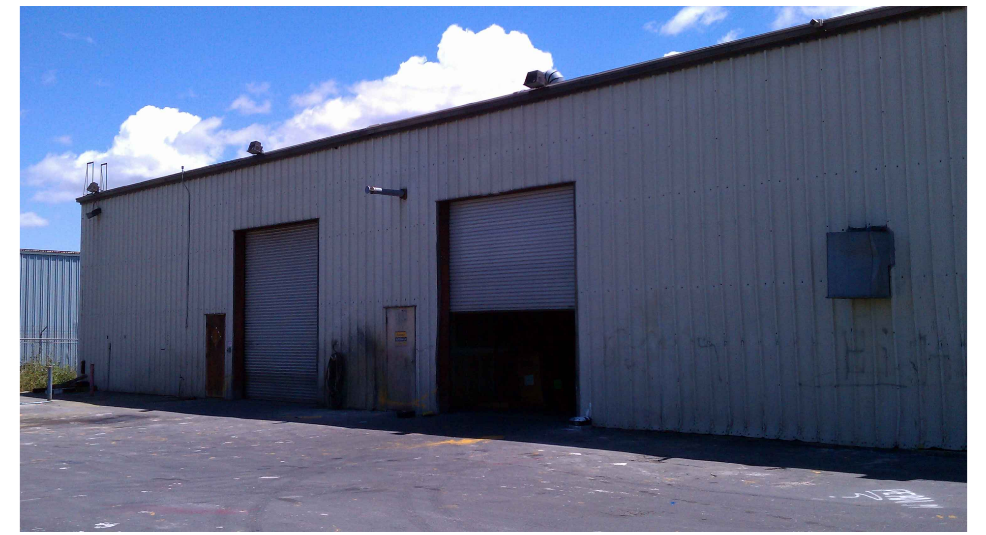
1 VIEW OF EXISTING METAL INDUSTRIAL BUILDING FROM KELLY COURT
