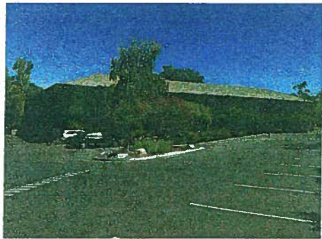
3 NW CORNER OF 2200 SAND HILL ROAD BUILDING SCALE: NTS E3.0
