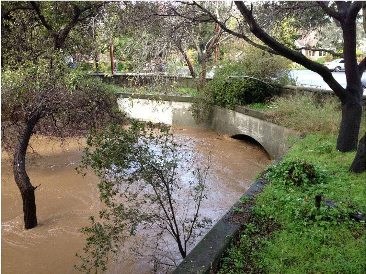
Figure 2 – Existing Culvert at Pope/Chaucer
