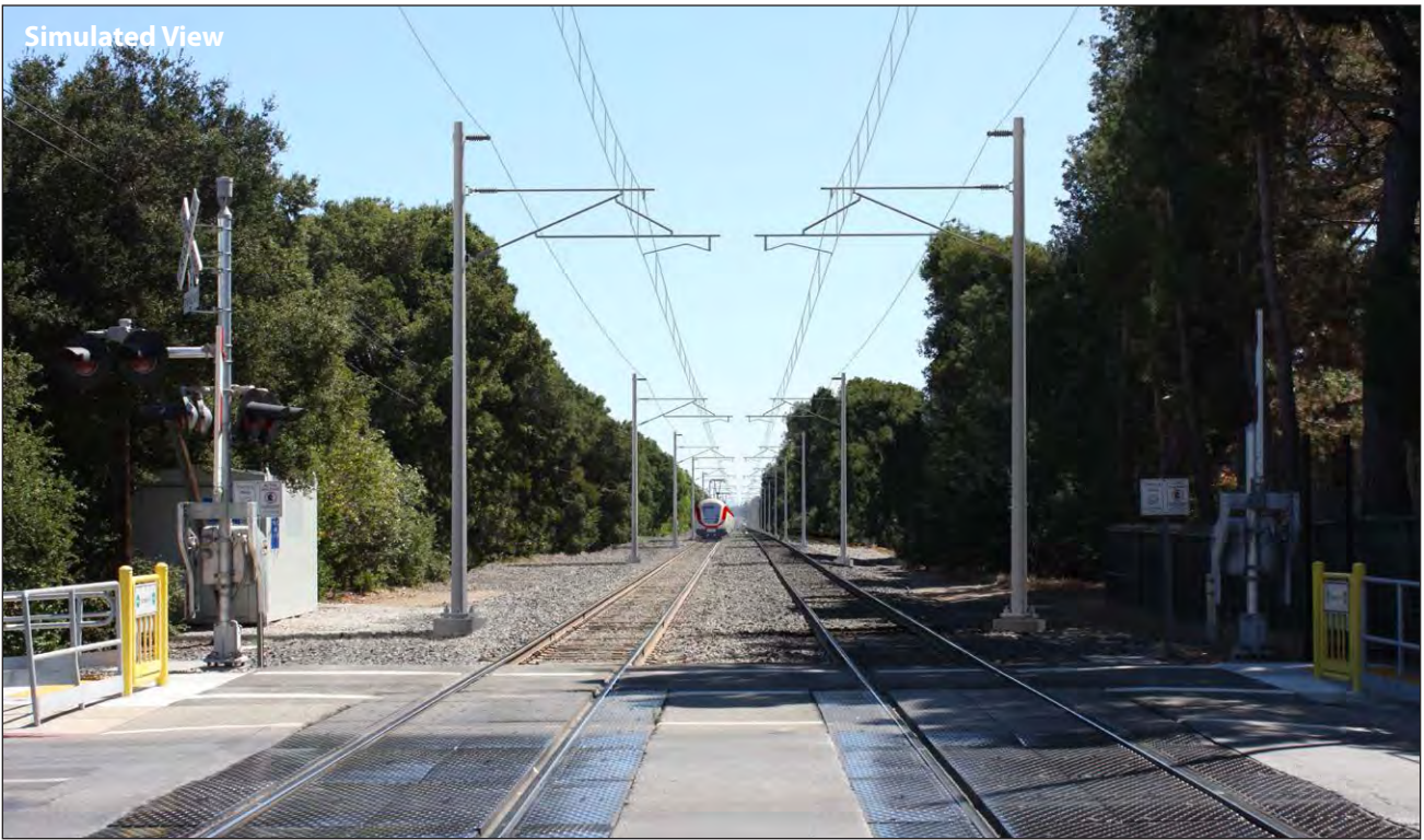
Looking southeast down the rail corridor with the OCS system and tree trimming, as seen from Churchill Avenue.
