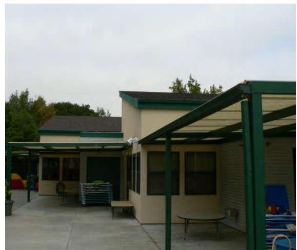
Figure 9 shows a view of Sections 1 and 2, which are on a shingle roof that is pitched at about 12°
