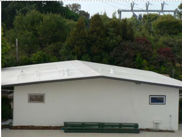
Figure 13 shows a view of the Teen Center rooftop, which includes Section 11 and Section 12
