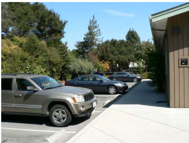
Figure 18 view of Section 1 carport area
