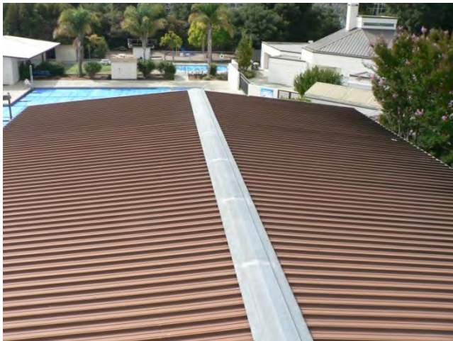
Figure 11 shows a view of Sections 7 and 9, which are metal standing seam
