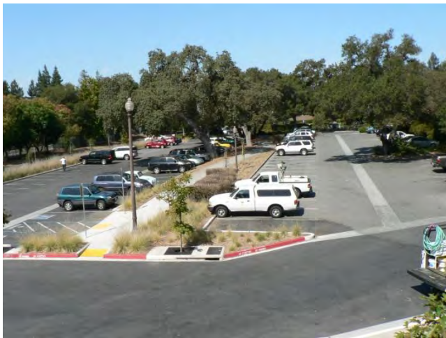
Figure 5 shows a view of the usable carport area
