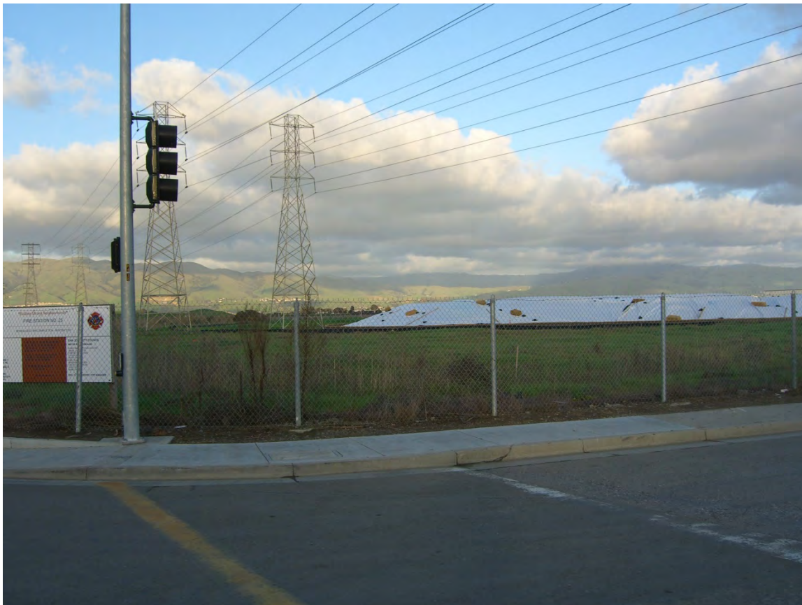
Fire Station 25: Looking from corner of Grand and Wilson.
