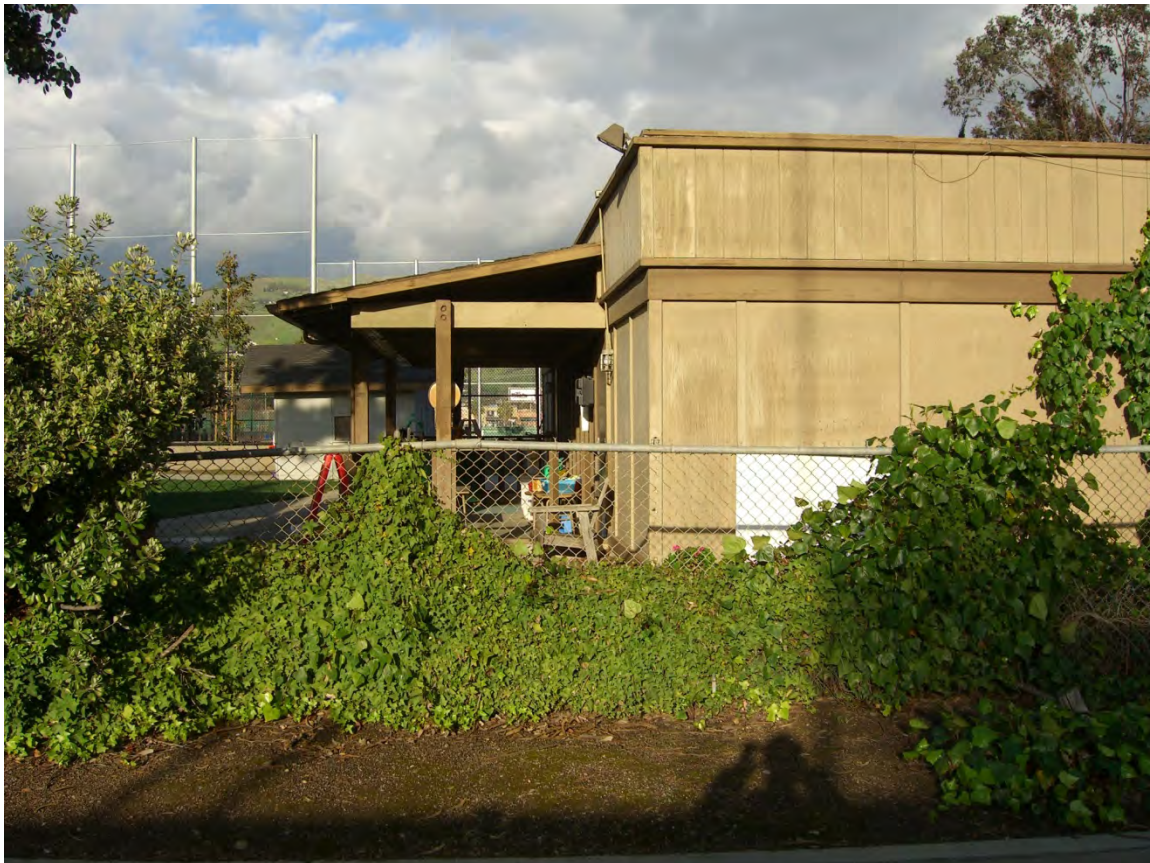
Fire Station No. 2: Day care center east of Fire Station 2, 54 ft. from proposed generator to the existing playground of day care facility.
