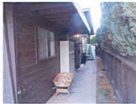
EXISTING FIRE STATION - TO BE DEMOLISHED - SOUTH SIDE YARD ELEVATION
