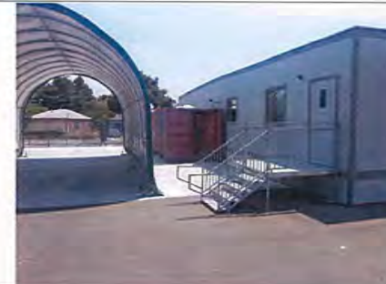
TEMPORARY FIREFIGHTERS QUARTERS & APPARATUS BAY
