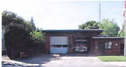
EXISTING MENLO PARK FIRE STATION #6 - TO BE DEMOLISHED - OAK GROVE AVENUE ELEVATION
