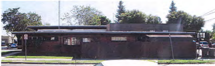
EXISTING MENLO PARK FIRE STATION #6 - TO BE DEMOLISHED - HOOVER STREET ELEVATION
