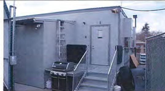
TEMPORARY FIREFIGHTERS QUARTERS & APPARATUS BAY
