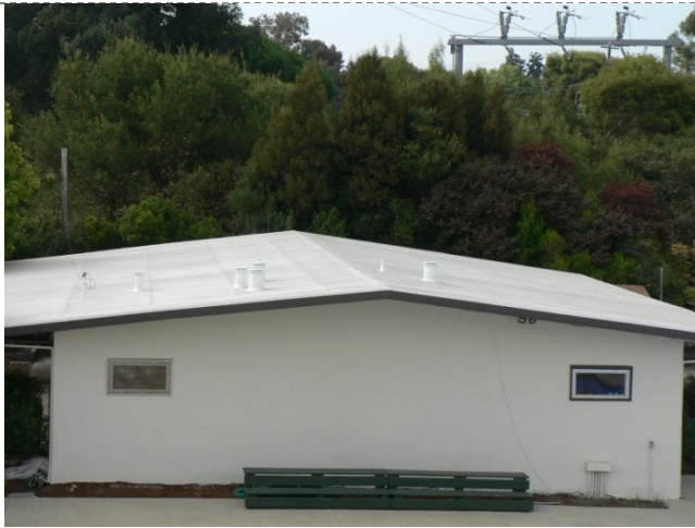
Figure 13 shows a view of the Teen Center rooftop, which includes Section 11 and Section 12
