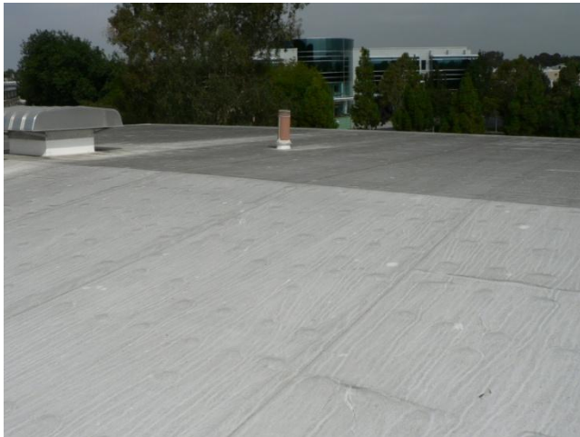
Figure 14 shows a view of Section 6, which is the highest area of the Community Center rooftop
