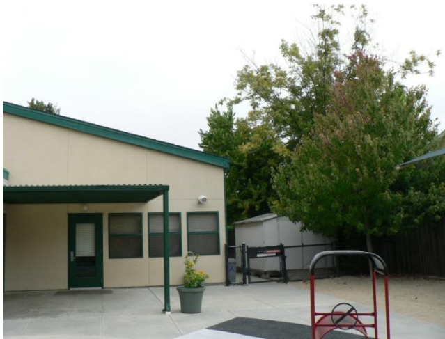
Figure 8 View of the tree that limits the usable area for Section 4
