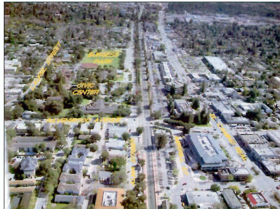
PHOTO 4 - VIEW OF RAVENWOOD AVENUE
