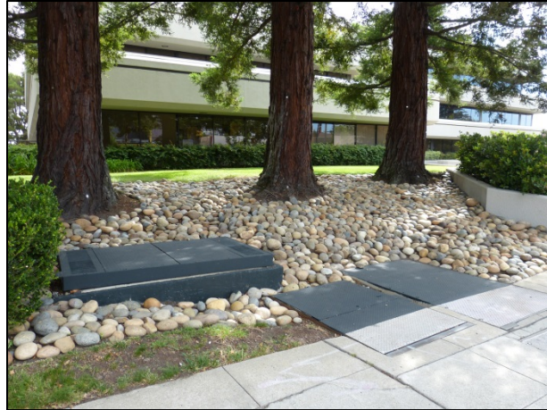
Photo 4. Coast redwoods #282 (right), 283 (center) and 284 (left). Note large utility vaults.
