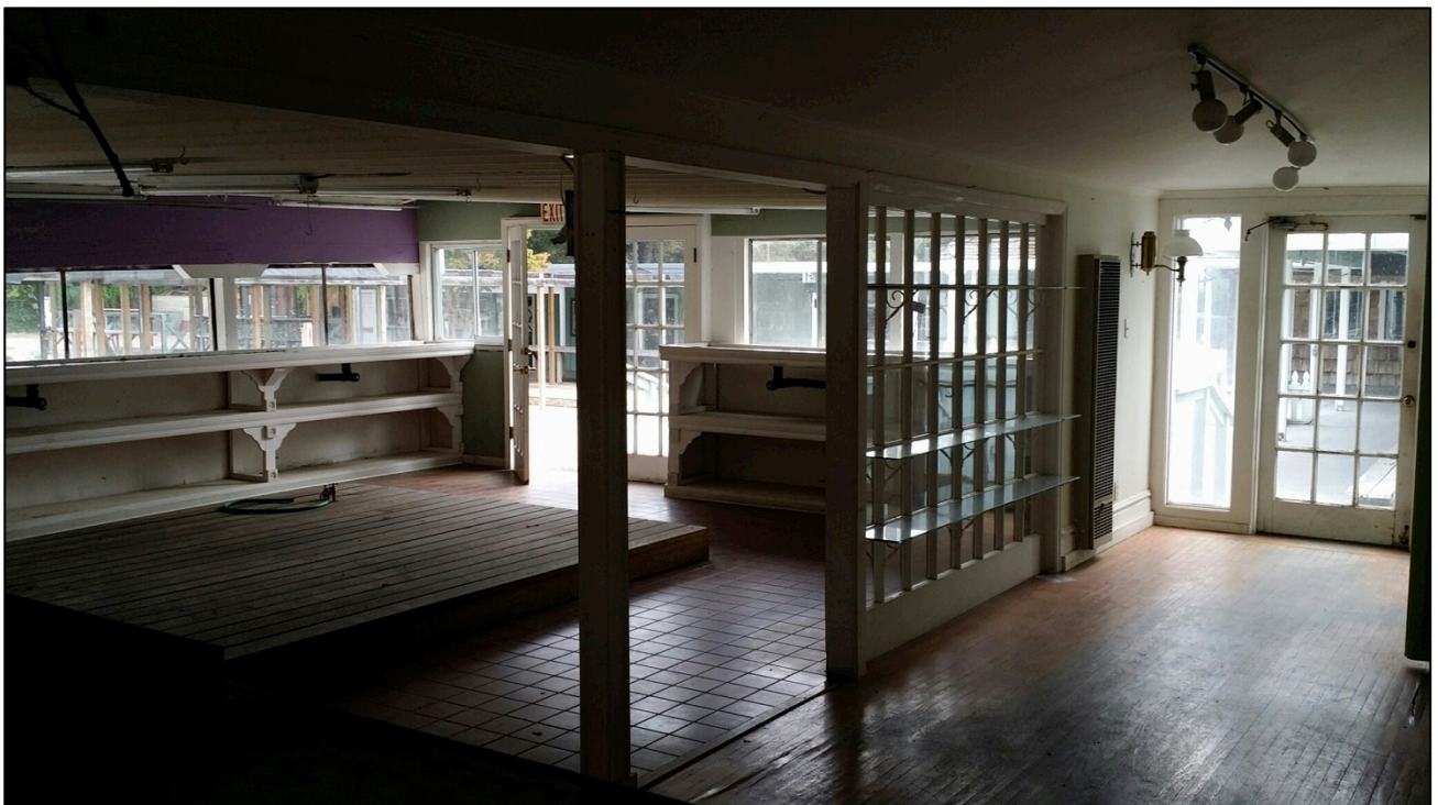
Carriage Stop, interior shops, looking north.
