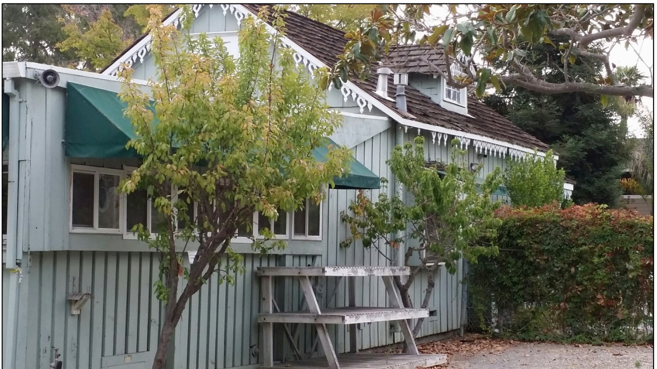
Carriage Stop, side elevation with roof dormer and rear addition, looking southeast.
