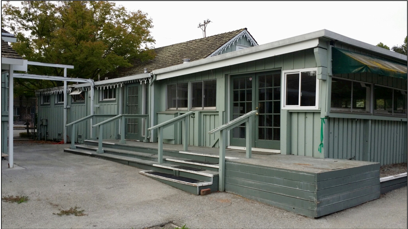
Carriage Stop, rear addition facing courtyard, looking southeast.
