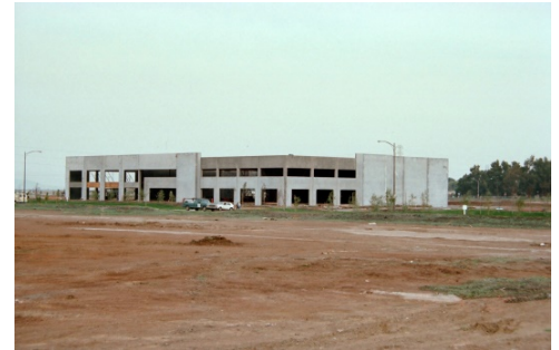
Office construction in the 1980s
