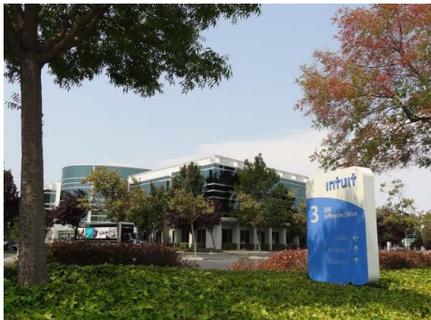
Offices originally constructed for Intuit
