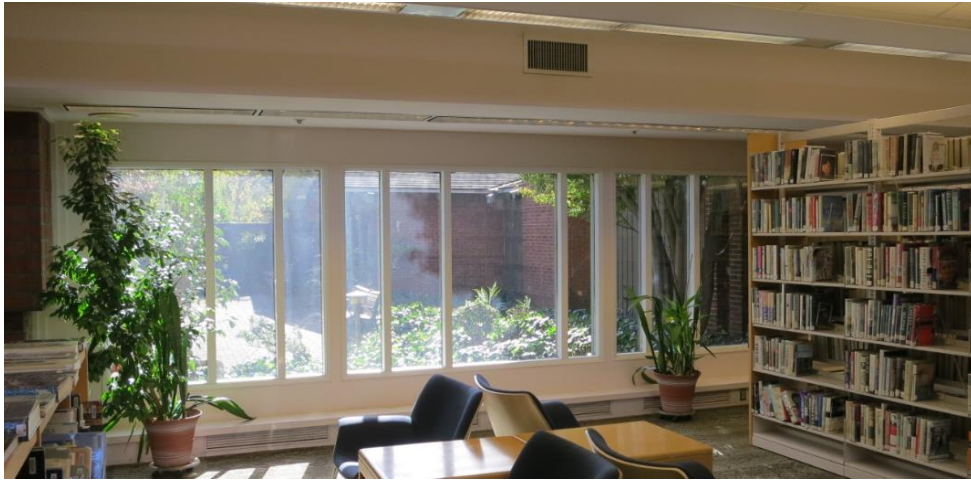
Typical Circulation Area – Note Supply Air Grille at floor.
