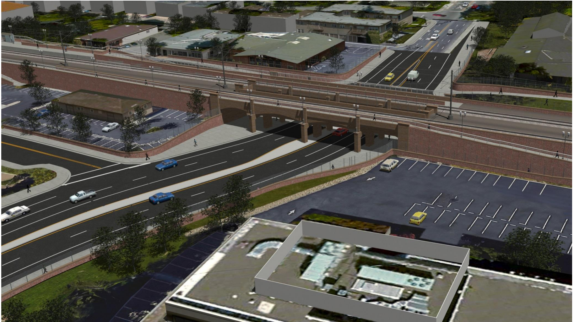
Ravenswood Avenue Railroad Crossing Project
