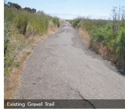
Existing Gravel Trail
