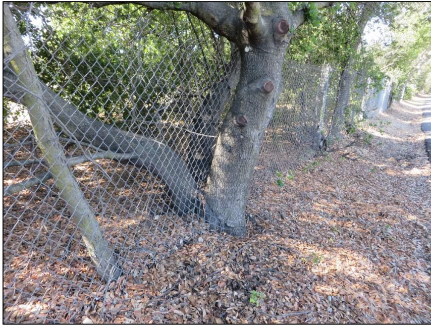
Photo 1 - Coast live oak #57 was embedded in the fence at a codominant attachment, increasing the likelihood for failure potential at that location.
