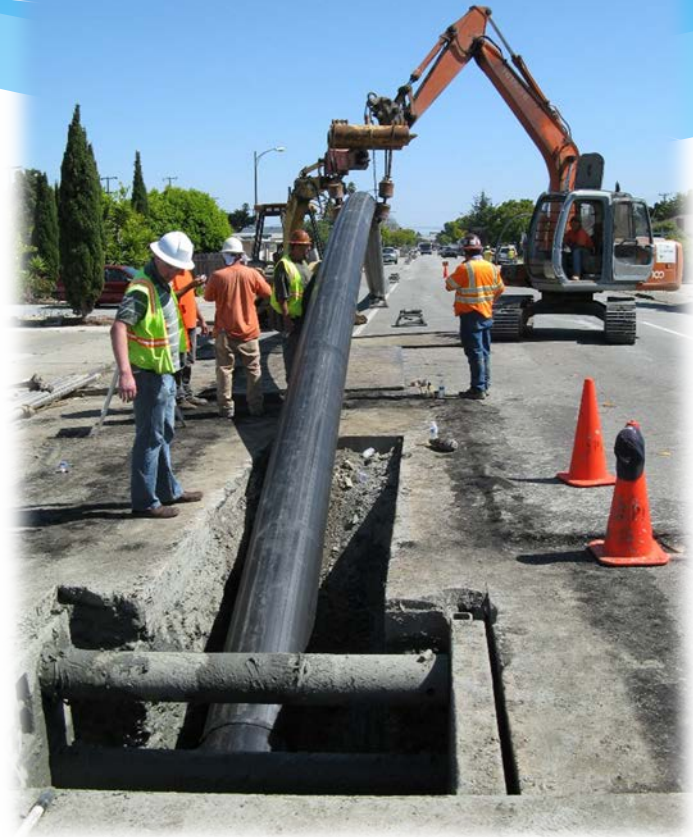
Trenchless: Horizontal Directional Drill (HDD)
