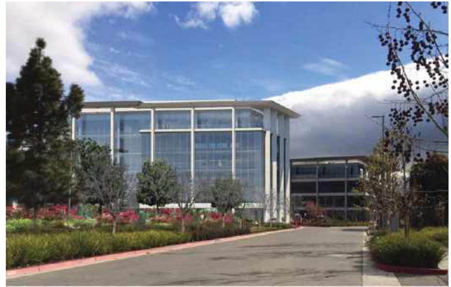
4 VIEW FROM PROJECT SITE LOOKING SOUTH
