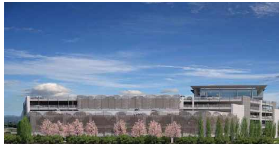
3 VIEW FROM EAST OF SITE LOOKING WEST
