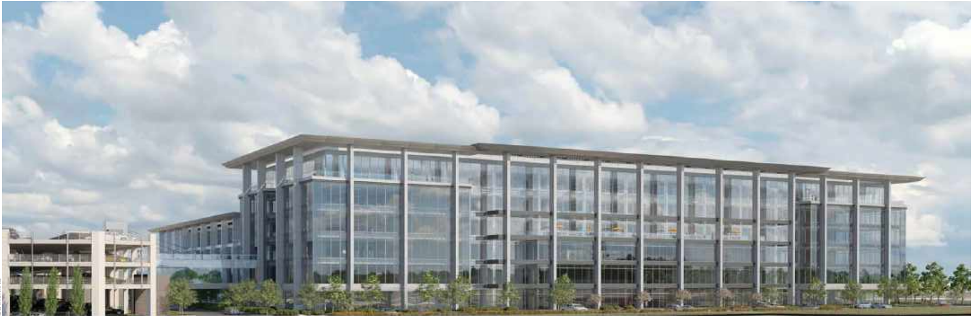
2 VIEW FROM NORTH OF SITE LOOKING SOUTH
