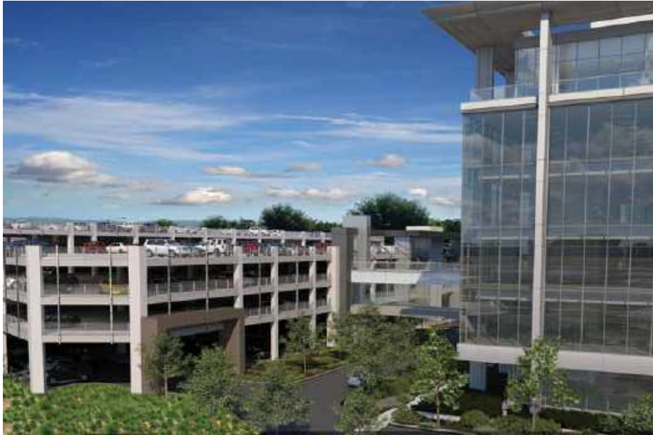
1 VIEW FROM NORTH OF SITE LOOKING SOUTH
