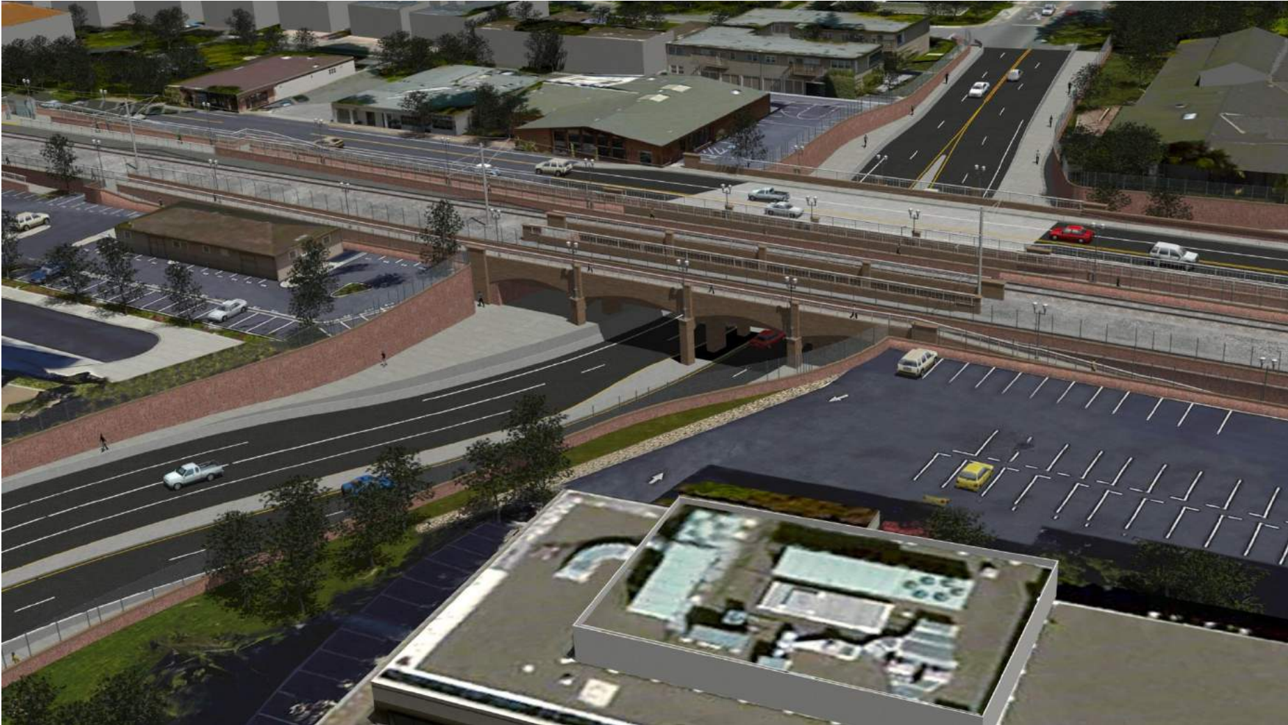
Ravenswood Avenue Railroad Crossing Project
