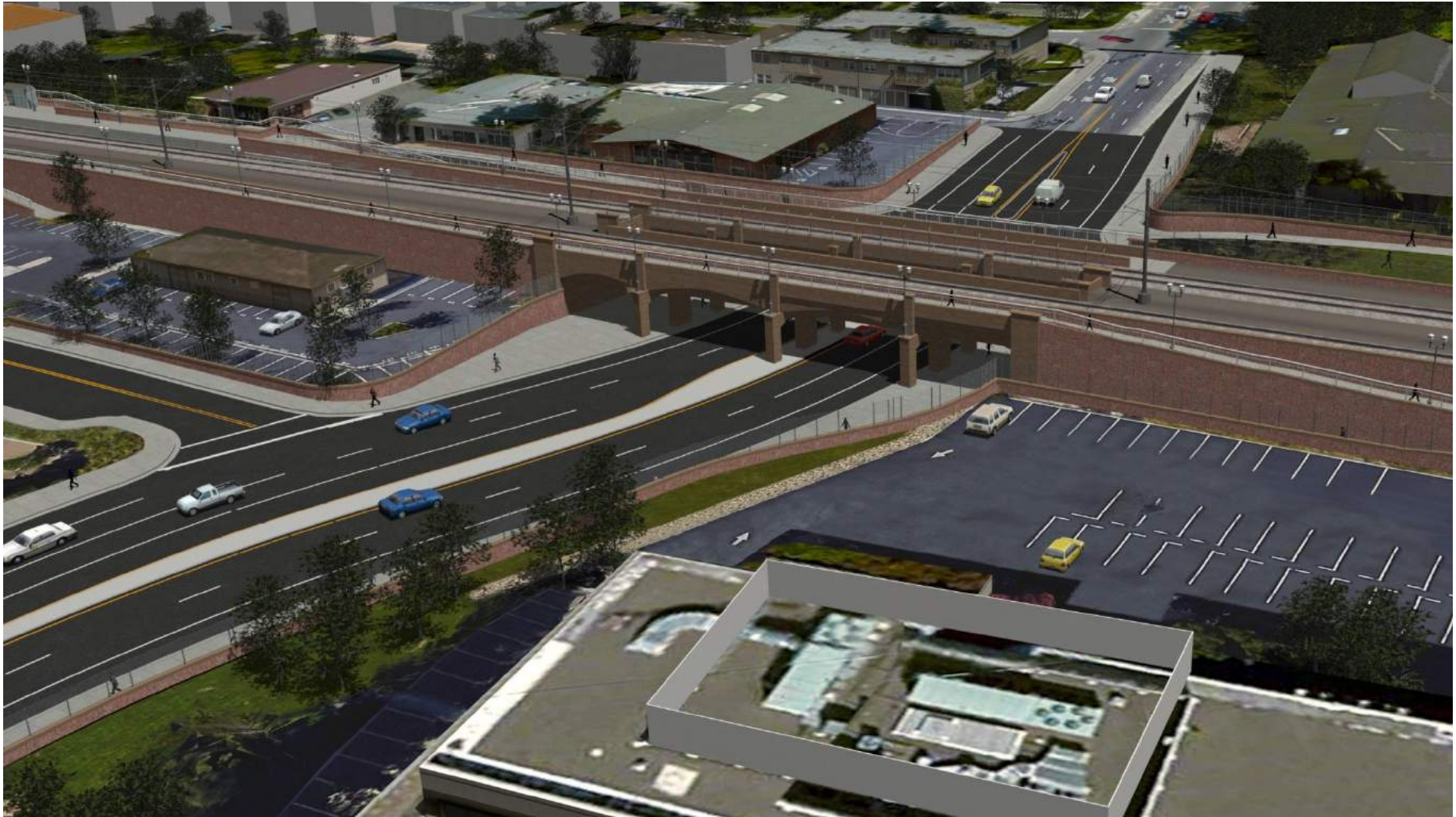
Ravenswood Avenue Railroad Crossing Project
