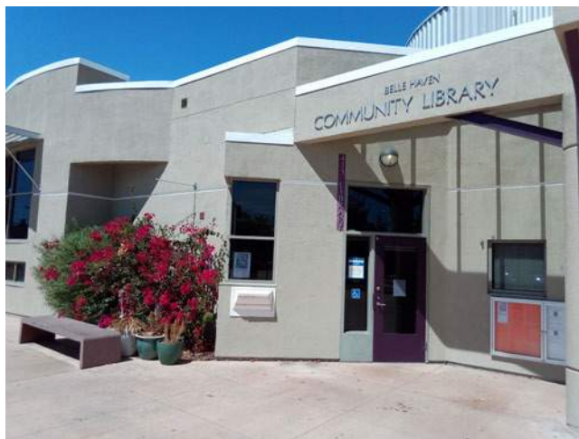
Exterior of existing Belle Haven Branch Library
