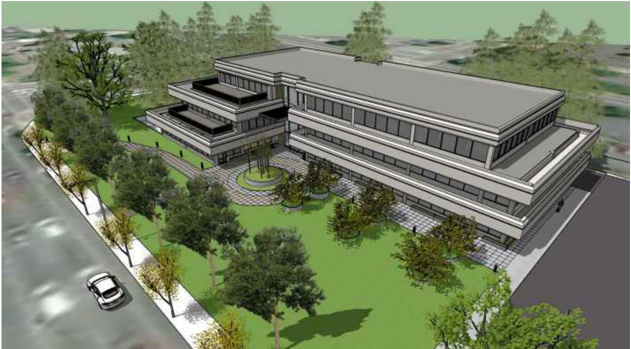
A-1.13 Aerial view of the property from above El Camino following completion. Trees near the building are encased in large planters located on top of structural columns in the garage below.
