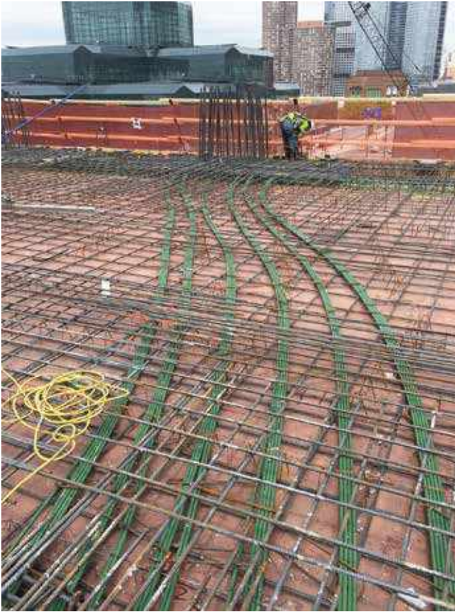
Fig. 4: Layout of post-tensioning and nonprestressed reinforcement
