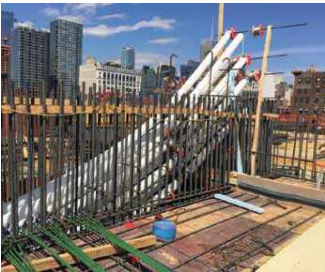
Fig. 8: Partial view of construction at Level 8
