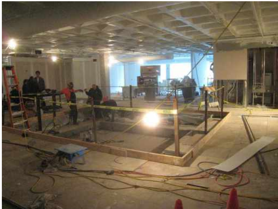
FIGURE 2 Work in progress
