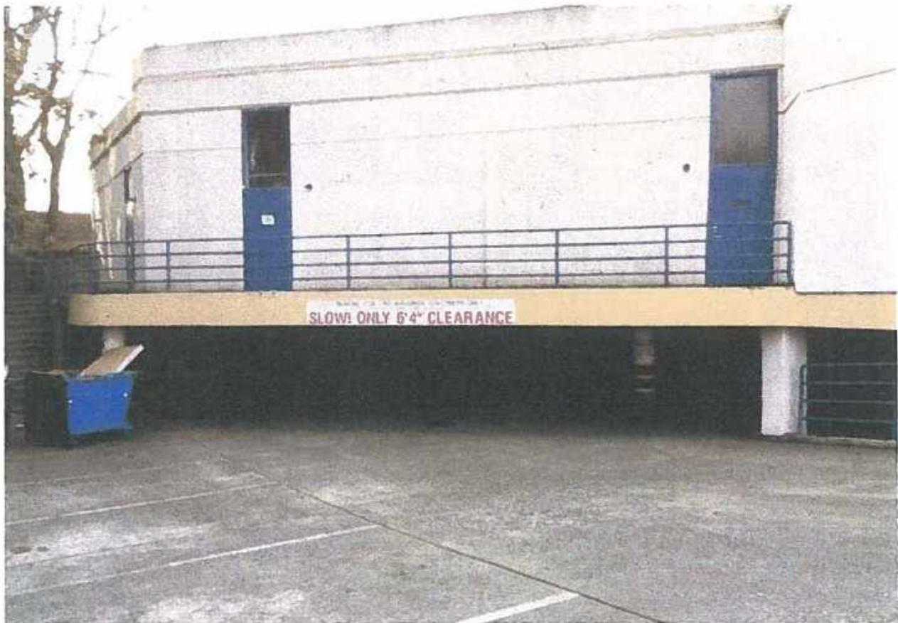
Figure 1. Below-grade parking at 1190 ECR (currently rented to Relax-the-Back and Fed-Ex), the property was re-developed 3 years after the property at 1000 ECR.
