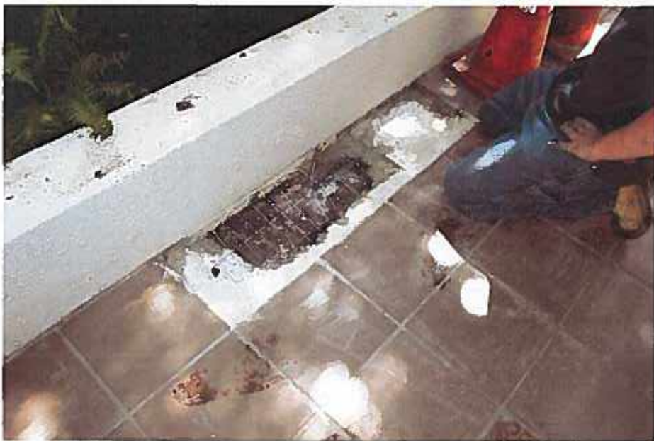
Figure 19 DT location at the walkway adjacent to the planter area.
