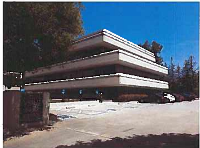
Figure 1 Menlo Park Office Center
