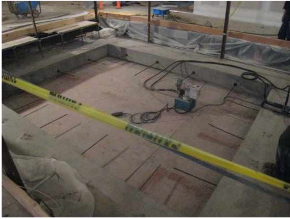
Figure 3 Tendons cut and re-anchored at the face of the opening
