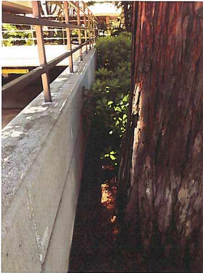
Photo 4 - Redwood trees close to the basement retaining wall
