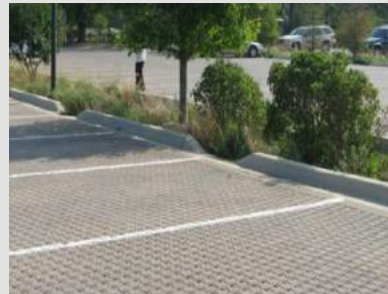
Example 2: Permeable paver w/ swale
