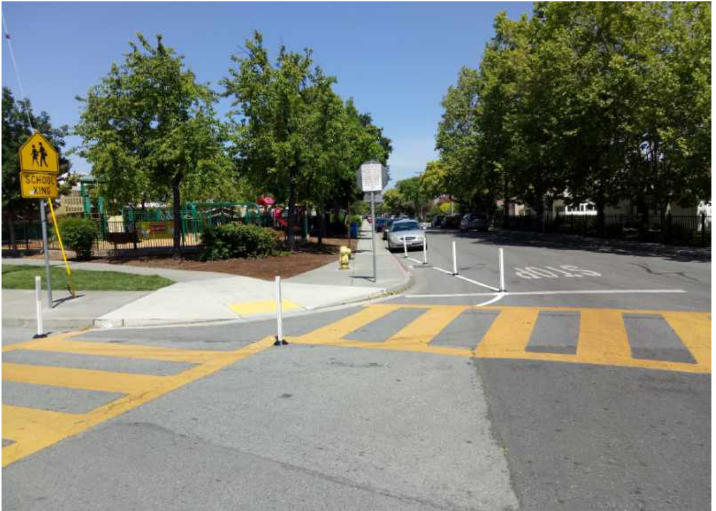
Sample trial bulbout at Chilco Street and Ivy Drive, Menlo Park
