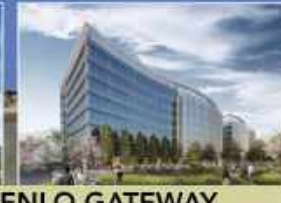
2 MENLO GATEWAY 105-155 Constitution Drive 495,052 SF Office Status: Under Construction
