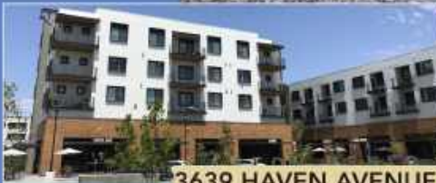
1 3639 HAVEN AVENUE St. Anton Partners 394 Apartments Status: Complete
