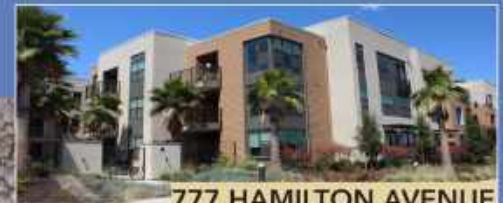
5 777 HAMILTON AVENUE Greenheart Land Company 195 Apartments Status: Complete
