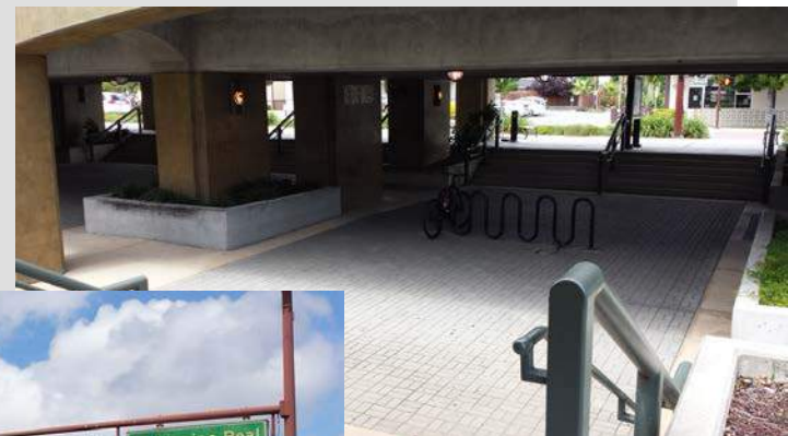
Plaza under station platform
