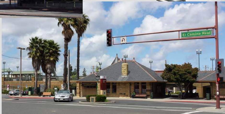
Main entrance on San Carlos Avenue and El Camino Real
