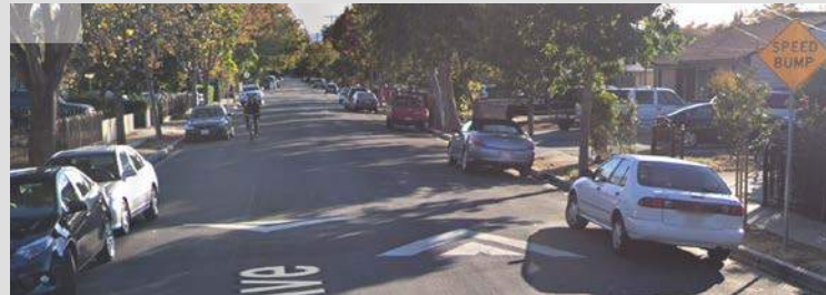
Speed Hump (Carlton Ave., Menlo Park)
