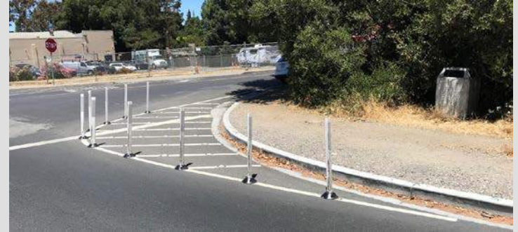
Bulbout (Middlefield Rd. and Woodland Ave., Menlo Park)
