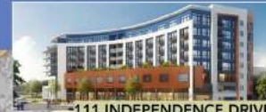
3 111 INDEPENDENCE DRIVE SP Menlo LLC 106 Multi-Family Dwelling Units Status: Pending Design Review
