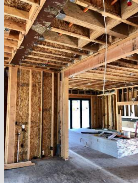
Typical Framing for One Wall Framed Construction
