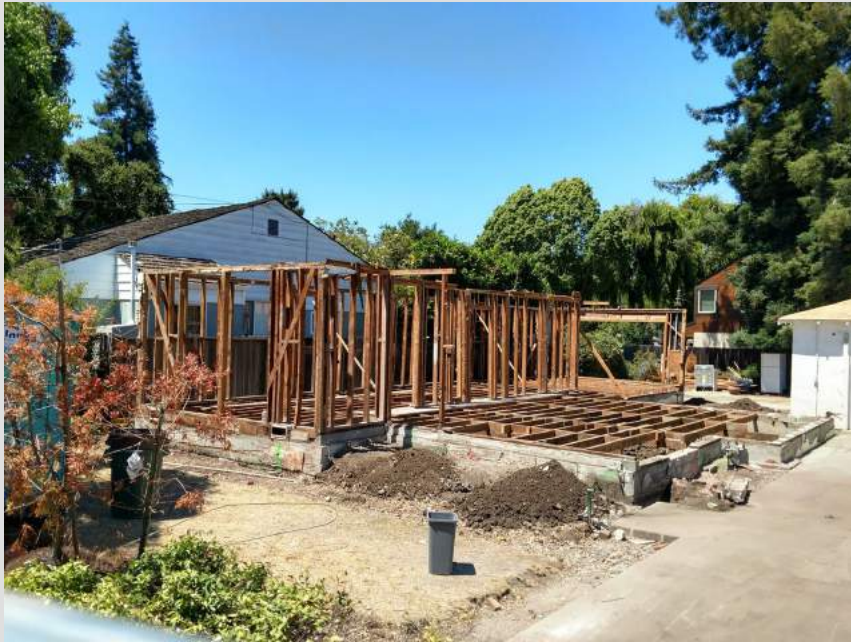
One wall Construction Alteration / Remodel
