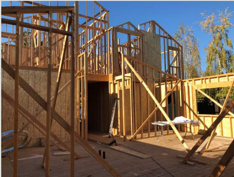
Typical New Construction Framing Over Existing Floors
