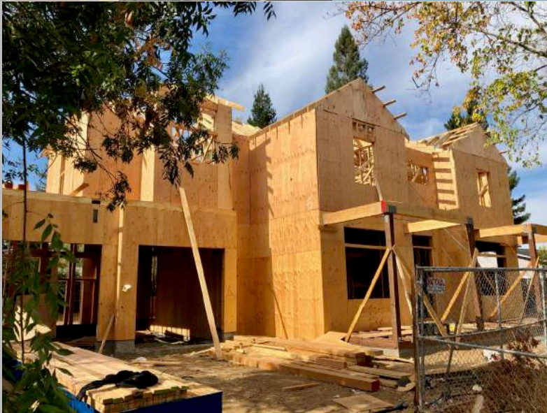
Typical New Construction Framing
