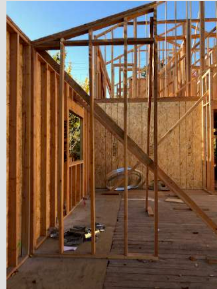
Typical New Construction Framing Over Existing Floors
