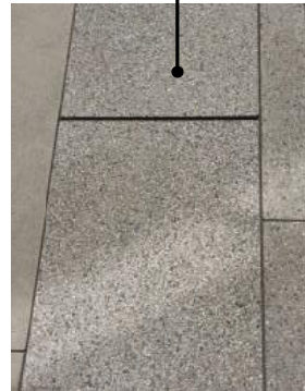
TYPE 4. CONCRETE UNIT PAVERS HEAVY SANDBLAST 24"X36"
