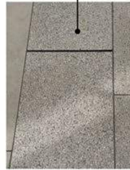
TYPE 4. CONCRETE UNIT PAVERS HEAVY SANDBLAST 24"X36"
