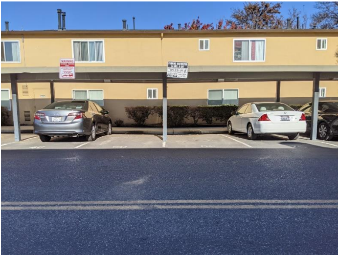
ADJACENT PROPERTY TO THE NORTH (MULTIFAMILY DEVELOPMENT)
