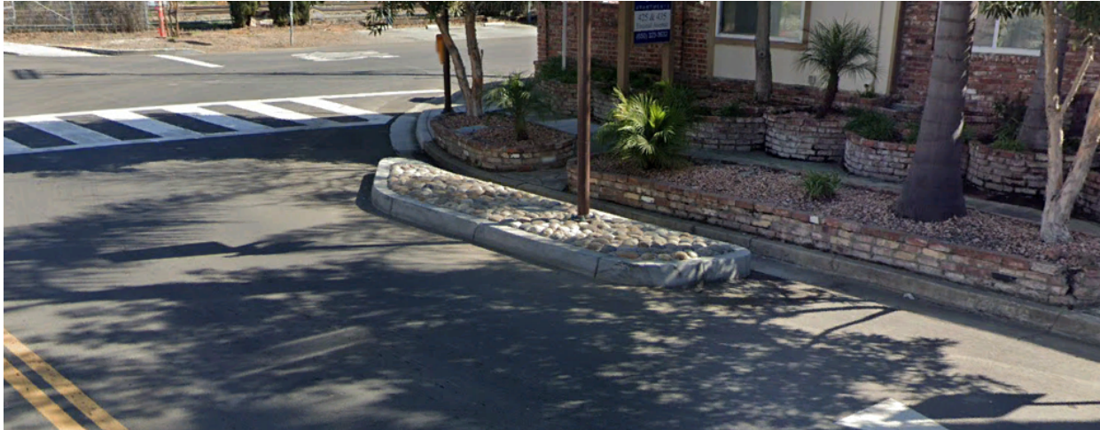
Example: Permanent detached intersection bulbout (Location: Encinal Ave. at Garwood Wy.)
